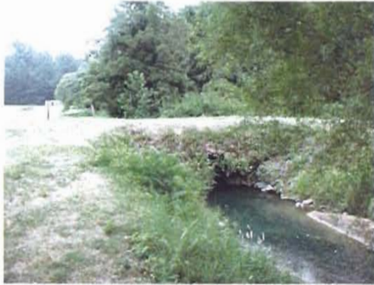
A. Footpath Crossing
