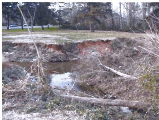
K. Bank Erosion on Silas Creek
