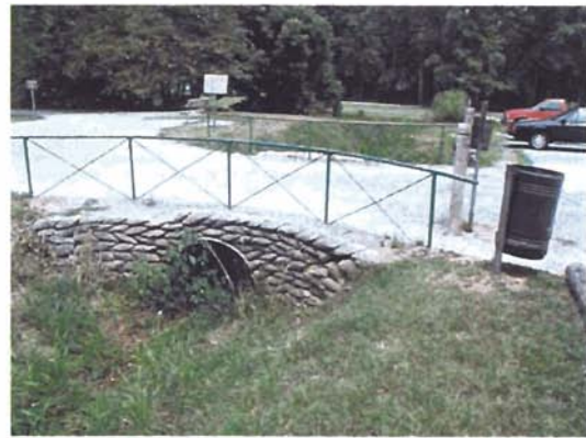
D. Bridge at Tributary on Reach 3
