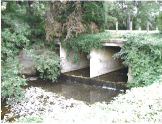
A. Culvert Downstream of Yorkshire Rd.
