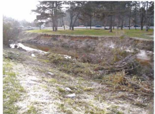
J. Bank Erosion on Silas Creek
