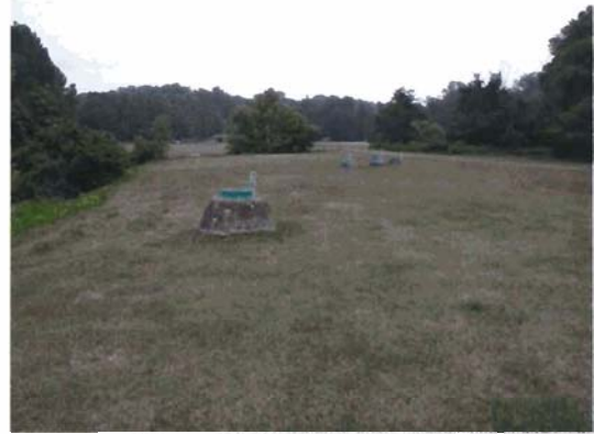
H. Sewer Lines on Left flank of Reach 2
