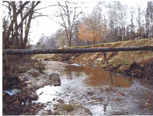
I. Bank Erosion on Silas Creek
