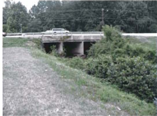
N. Culvert Upstream of Silas Parkway
