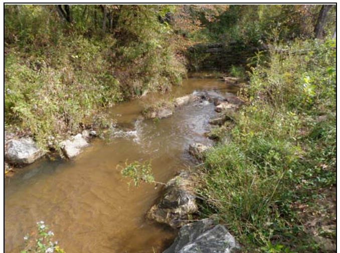
M4 Photo Point 2 – Problem cross-vane at station 66+75
