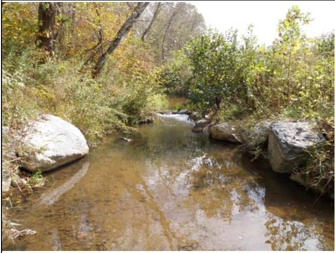
M4 Photo Point 3 – Problem cross-vane at station 63+50
