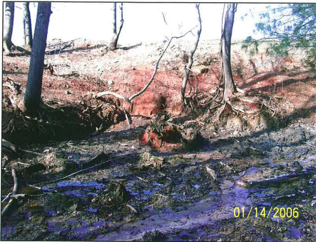
15. Cattle intrusion was also noted along the upstream portion of the Unnamed Tributary in an area where the valley broadens, causing extreme degradation of the bed and banks and denuding of vegetation.
