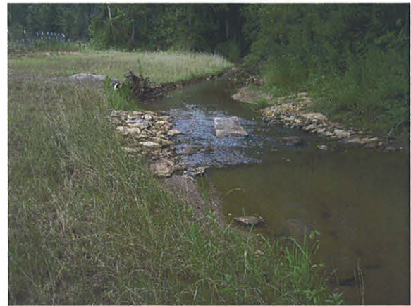
Photograph No. 16- Dual Winged Jetty With Boulder Cluster and Root Wad 1 Looking Downstream
