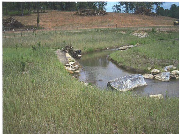
Photograph No. 8- J-Hook 3 Looking Downstream
