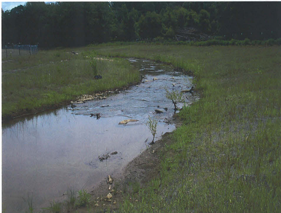
Mainstem Reach – Constructed Riffle – Downstream End – Over Tightened Meander
