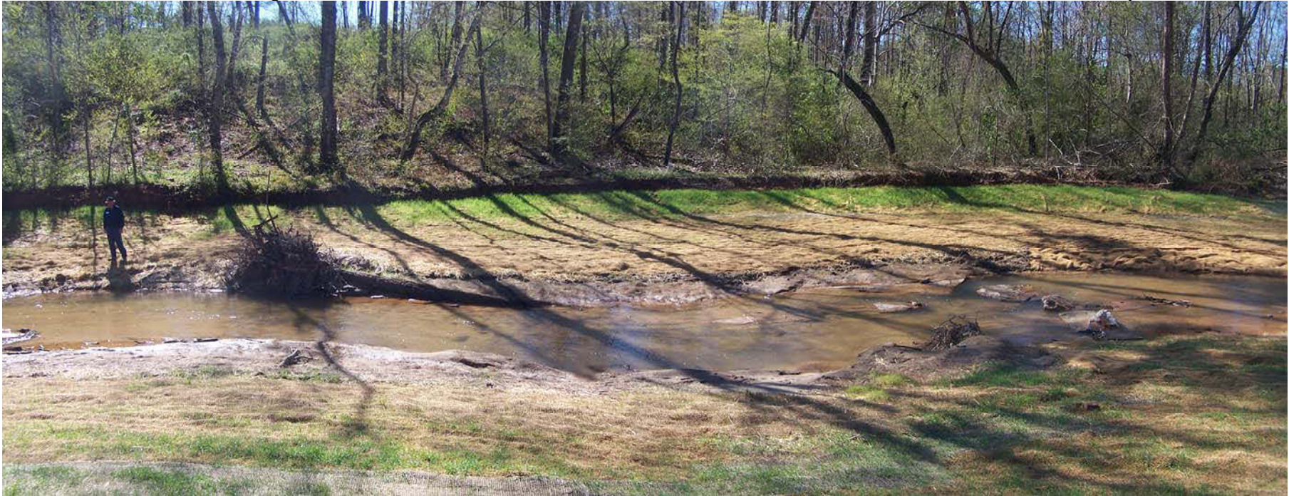
Mainstem Reach – Log-Vane, J-Hook, Root Wad Combination Structure – After Herbaceous Ground Cover Established – April 2007
