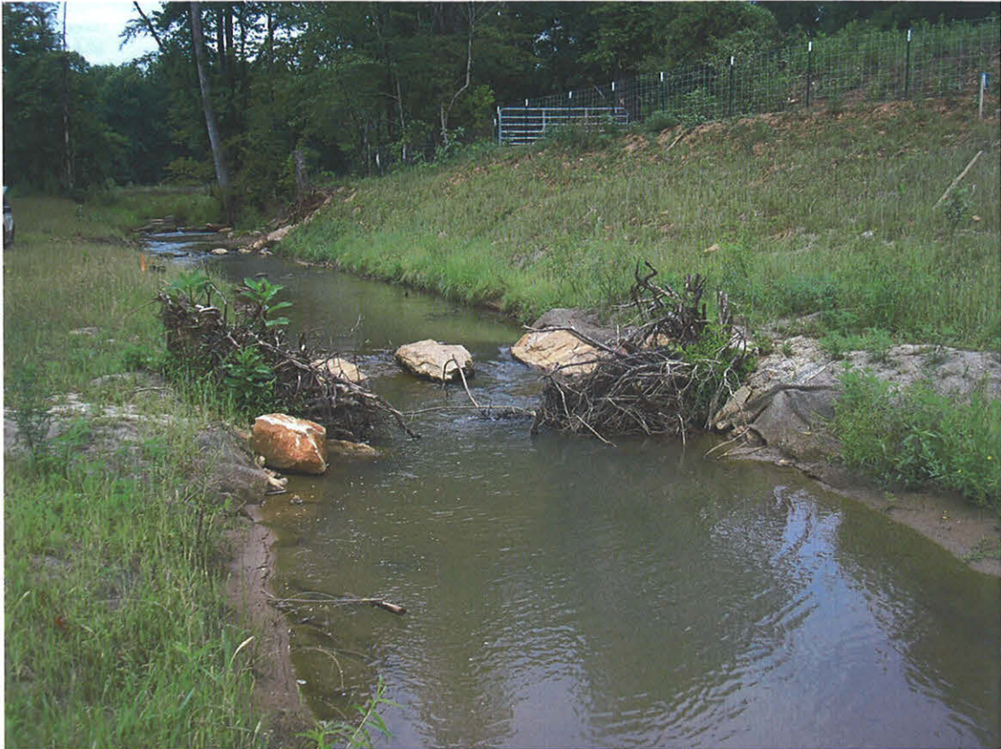
Mainstem Reach – Cross-Vane No.1 - Post Revetment – Looking Upstream
