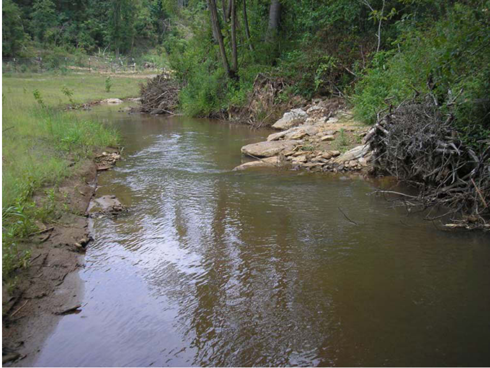
Single Arm Rock Vane with Root Wad Bank Stabilization (shown above) – Post-Restoration Looking Upstream
