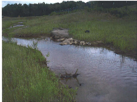
Photograph No. 4- Rock Vane 1 Looking Downstream
