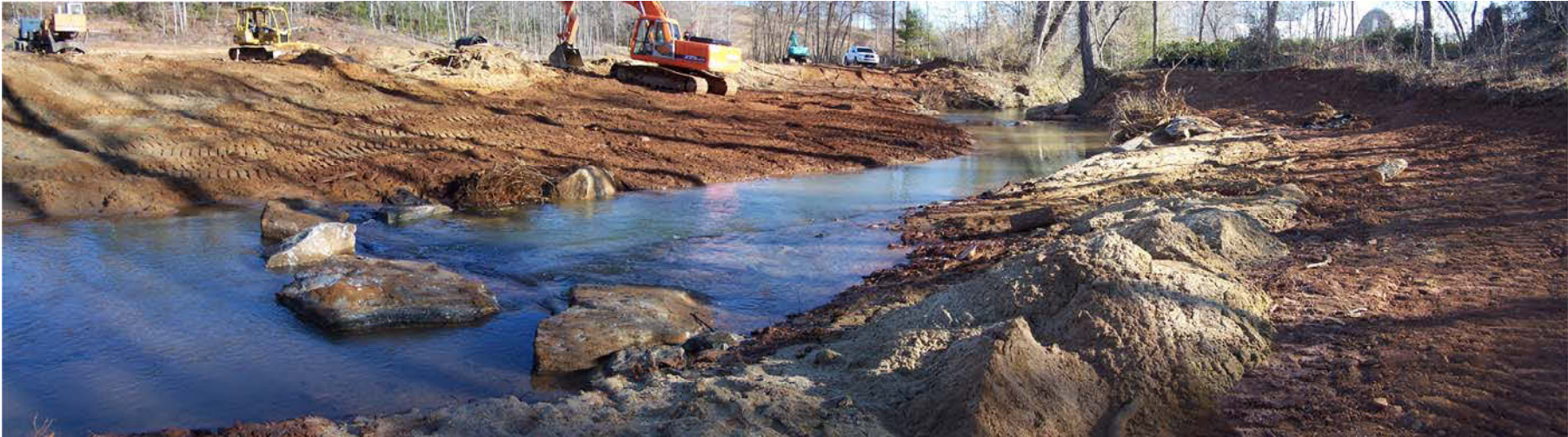
Mainstem Reach – Log-Vane, J-Hook, Root Wad Combination Structure – During Construction – February 2007
