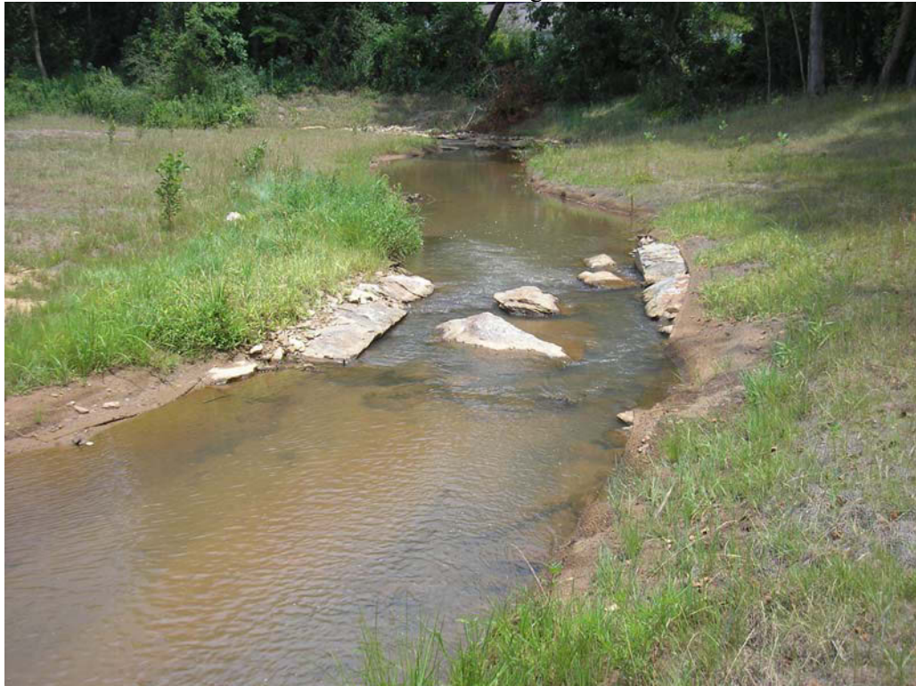
Rock Vane with Upstream Boulder Cluster – At confluence of UT-D – Looking Downstream
