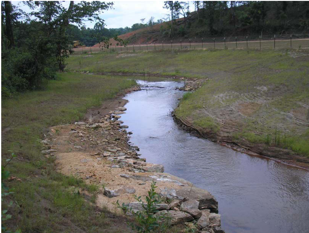
Single Arm Rock Vane above confluence of UT-C with Silver Creek Mainstem
