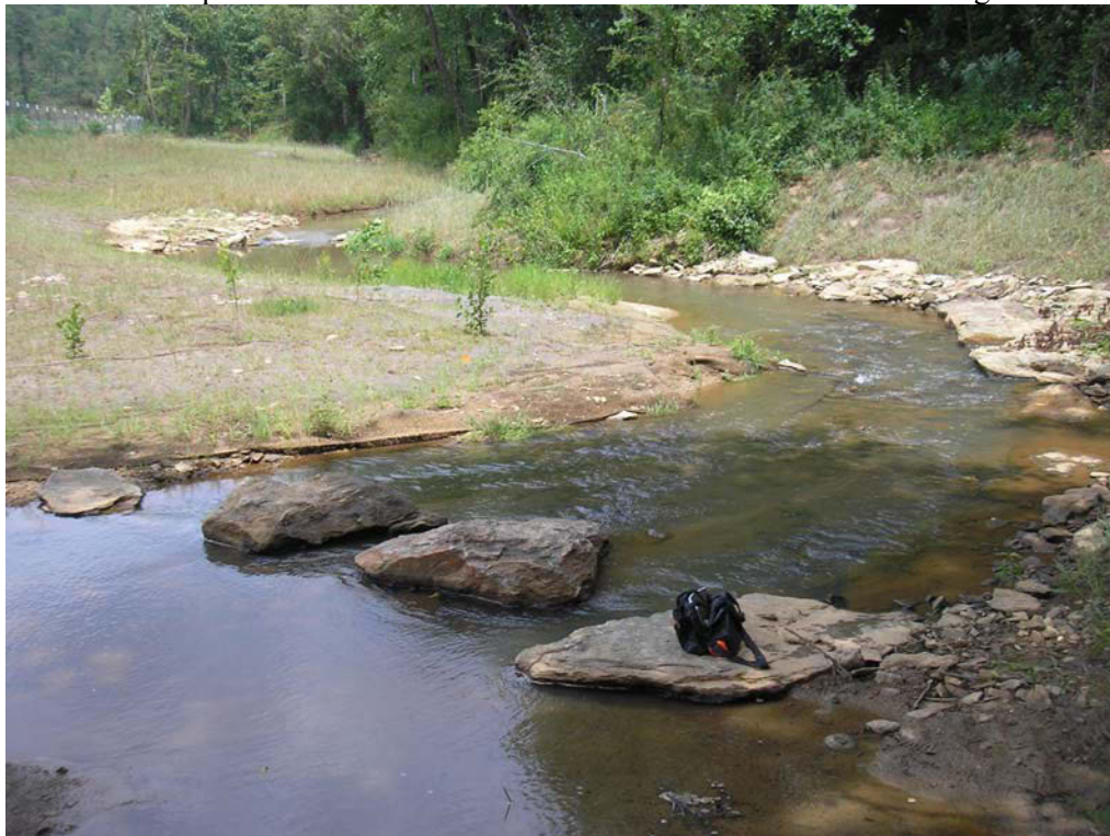
Rock Vane with Upstream Boulder Cluster – At confluence of UT-D – Looking Downstream
