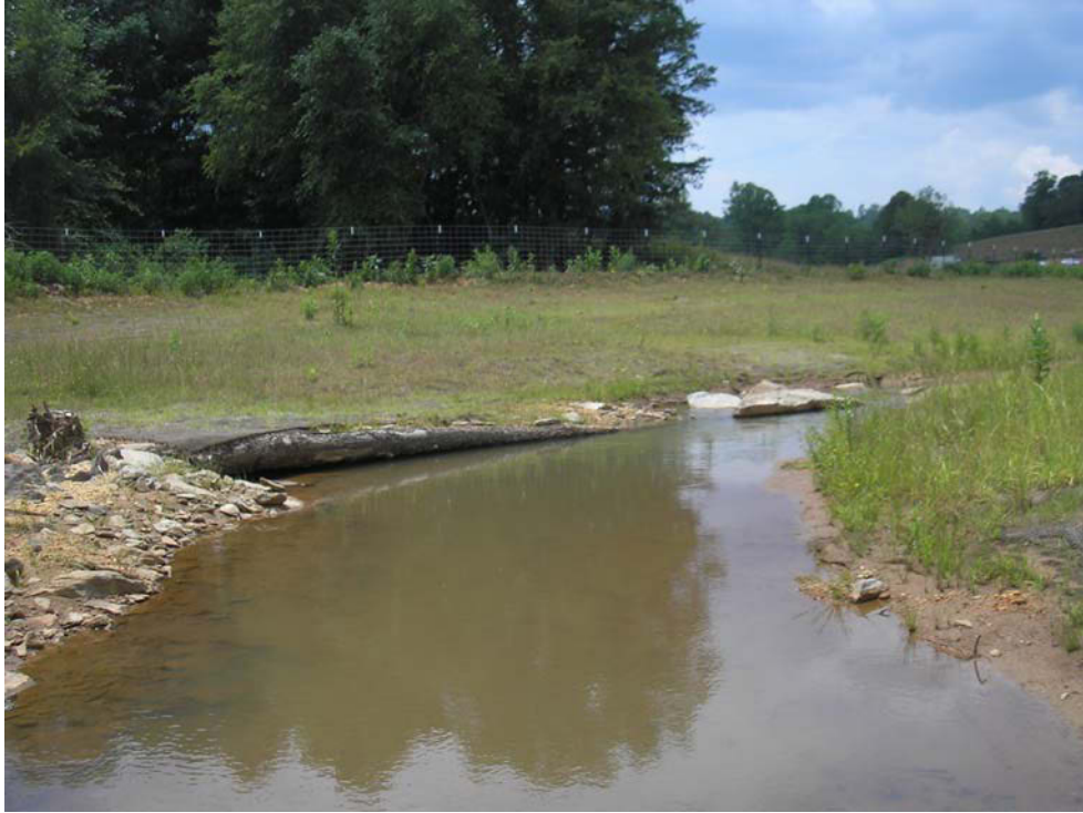
Log-Vane J-Hook Structure – Upstream from former Abandoned Oxbow – Post-Restoration - Looking Upstream
