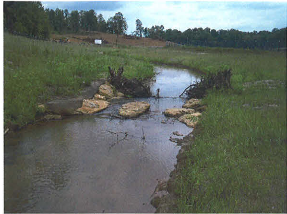
Photograph No. 2- Cross Vane 1 Looking Downstream
