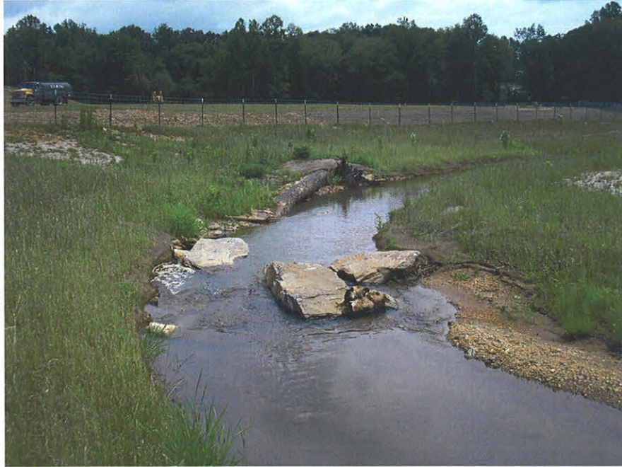
Mainstem Reach – Constructed Riffle – Downstream End – Over Tightened Meander
