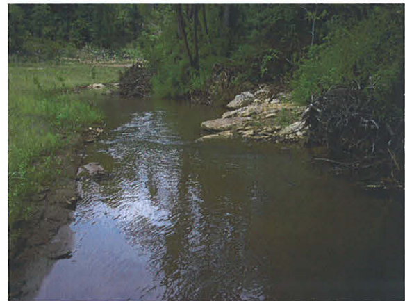
Photograph No. 18- Rock Vane 4 and Root Wad 3 Looking Downstream
