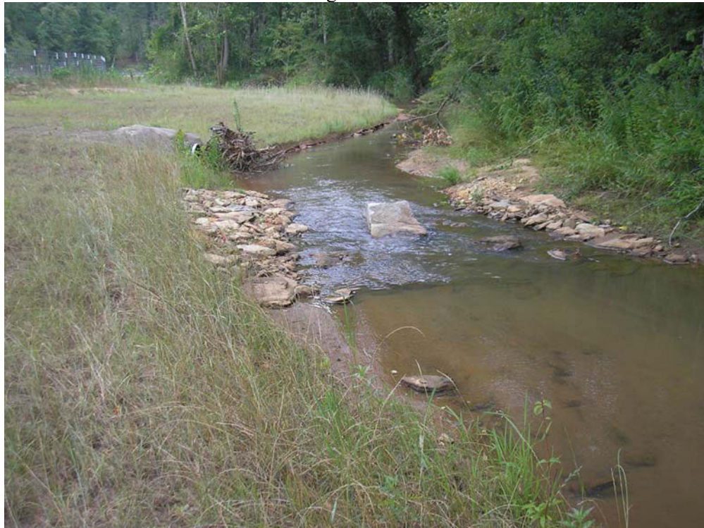
Dual Winged Jetty Riffle with Random Boulder Cluster – Downstream from confluence of UT-D – Looking Downstream
