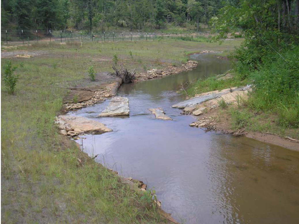
Rock Toe Channel Reinforcement upstream from confluence of UT-C with Mainstem – Post-Restoration Looking Upstream
