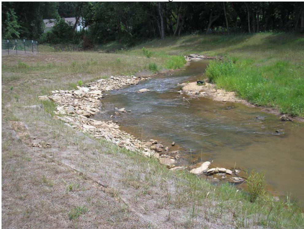
Constructed Riffle with Rock Toe Bank Reinforcement - Location of former Abandoned Oxbow Post Remediation – Looking Downstream
