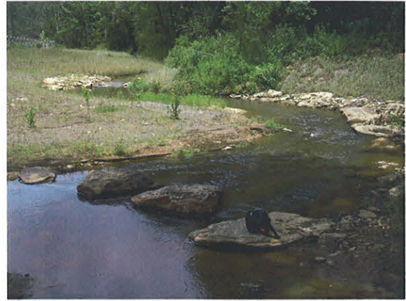
Photograph No. 14- Rock Vane 3 With Boulder Cluster Looking Downstream
