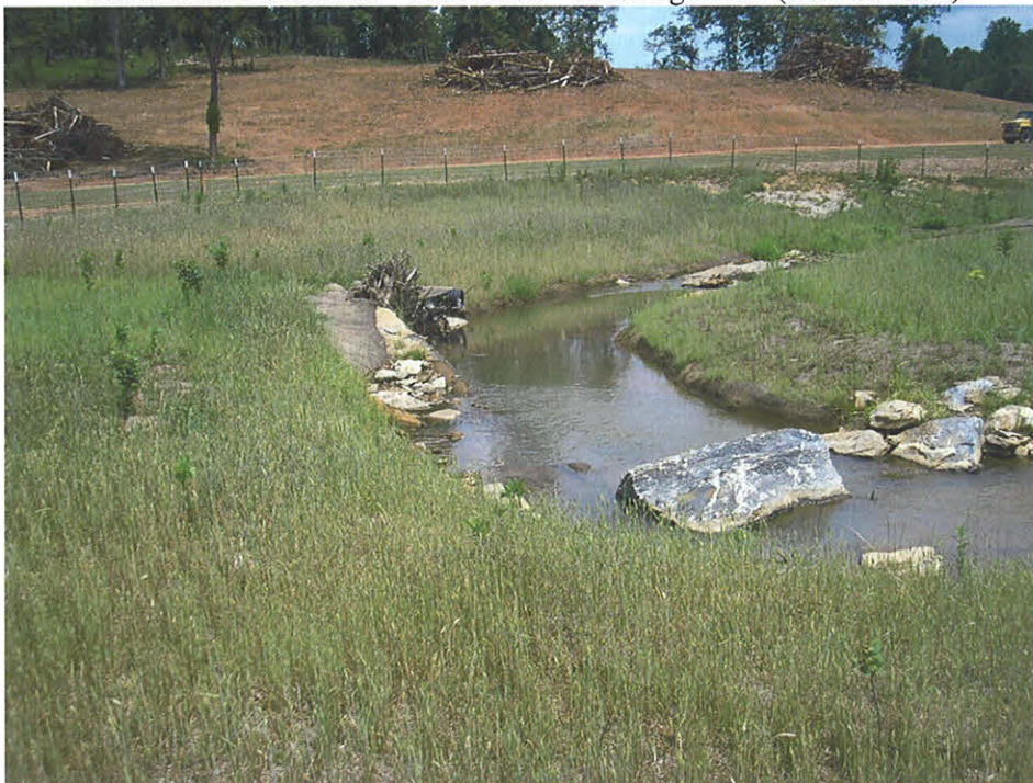
Mainstem Reach – Over Tightened Meander – Post-Restoration - Log Vane - J-Hook – Root Wad Combination Structure – Mid-Bend – Looking North (Downstream)
