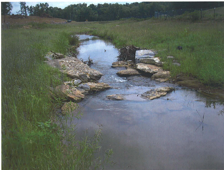
Mainstem Reach – Cross-Vane No. 2 – Post Restoration – Looking Downstream
