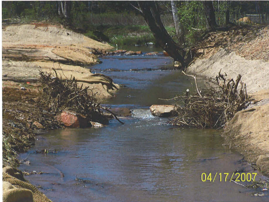
Mainstem Reach - Cross-Vane No. 1 with Root Wad/Boulder Cut-Off Sills, looking Downstream
