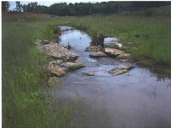
Photograph No. 3- Cross Vane 2 Looking Downstream
