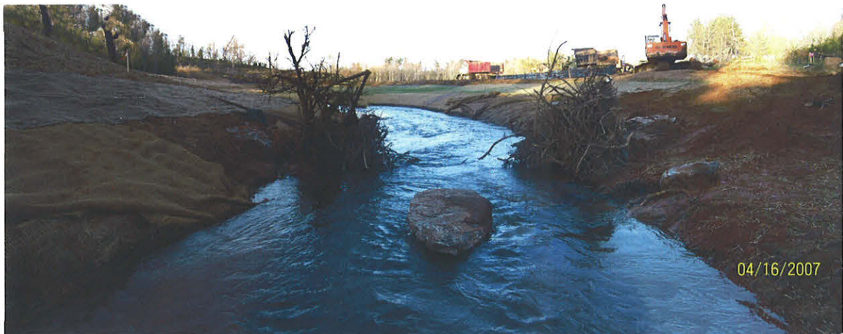
Mainstem Reach - Cross-Vane No. 1 with Root Wad/Boulder Cut-Off Sills, looking Downstream
