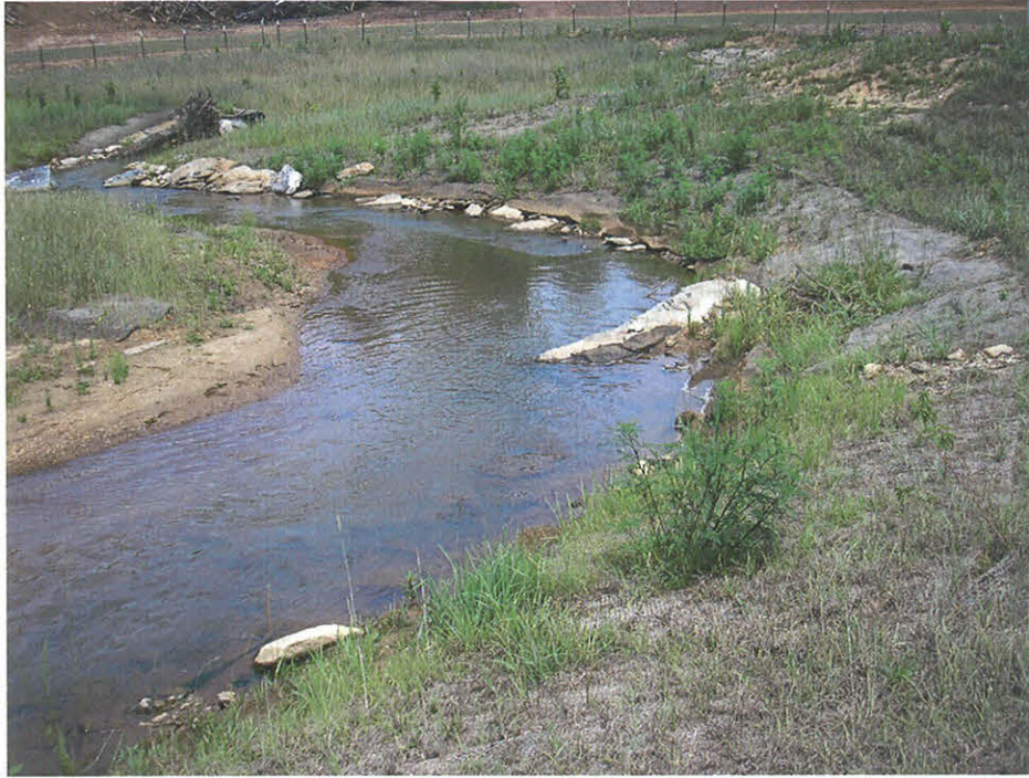
Mainstem Reach – Over Tightened Meander – Post-Restoration - Log Vane - J-Hook – Root Wad Combination Structure – Mid-Bend – Looking North (Downstream)
