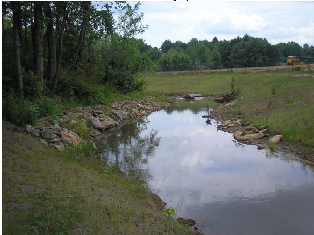
Rock Toe Channel Reinforcement upstream from confluence of UT-C with Mainstem – Post-Restoration Looking Upstream
