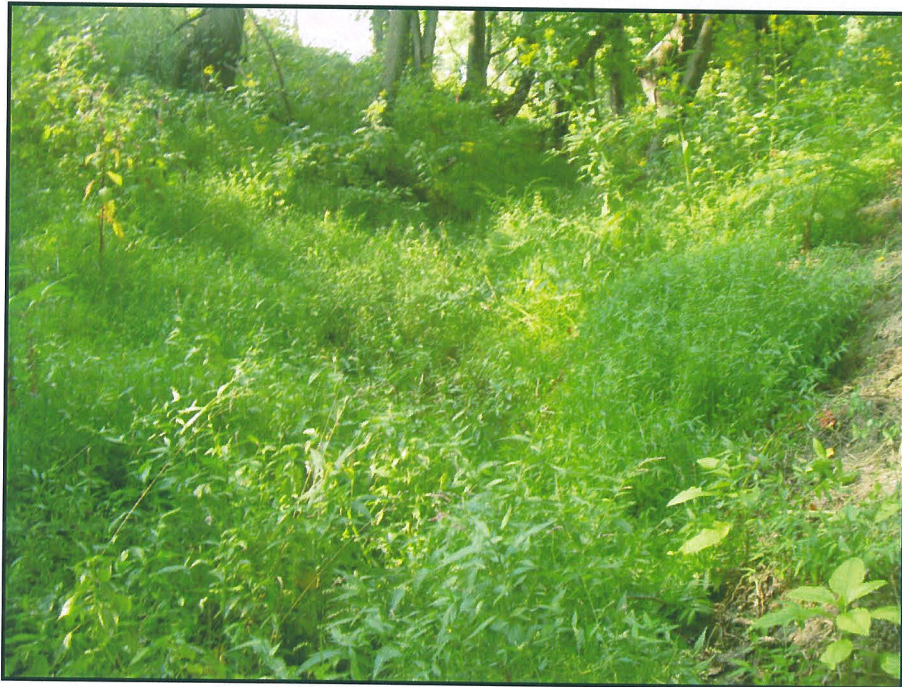
Fixed Station 8 Overview of UT-A, facing upstream near station 11+00. (EMH&T, September 8, 2008)
