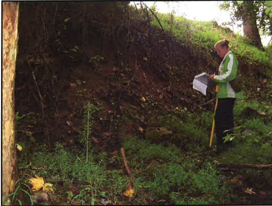
SPA 3 Vertical bank along Unnamed Tributary A near station 8+50. (EMH&T, Inc. 9/17/09)
