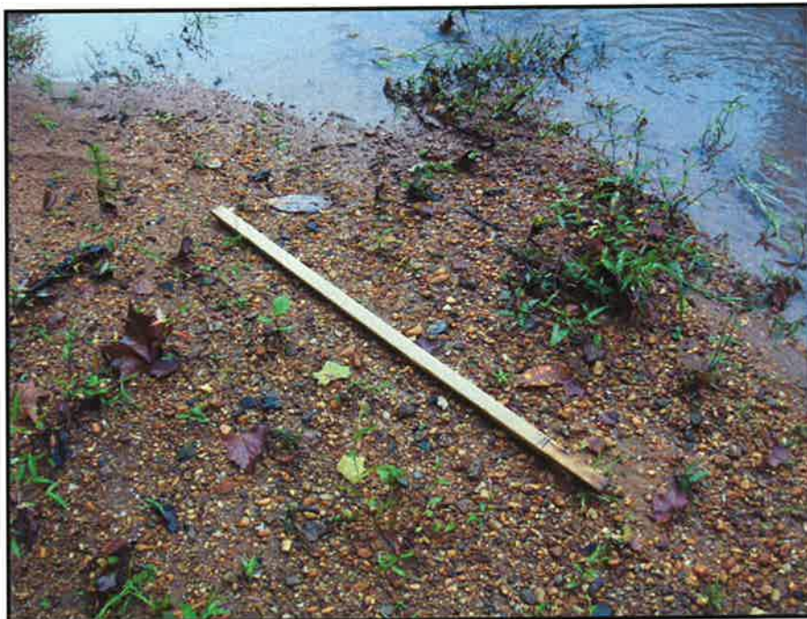
BF 2 Crest Gage on Silver Creek Mainstem (Year 3). (EMH&T, 9/21/09)
