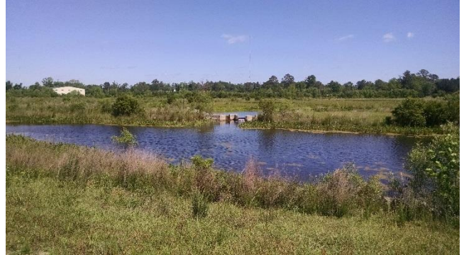
Outlet weir looking towards Cell D
