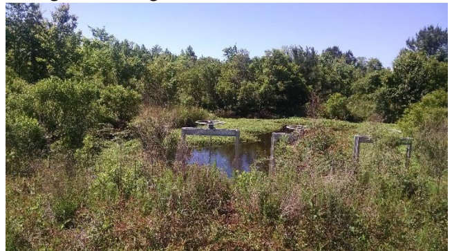
Tidal gates looking towards outlet
