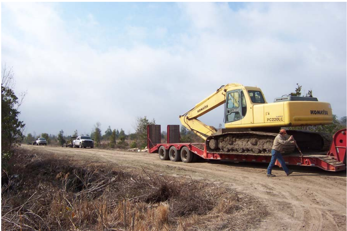
Heavy equipment used to install ditch plugs throughout wetland restoration area.
