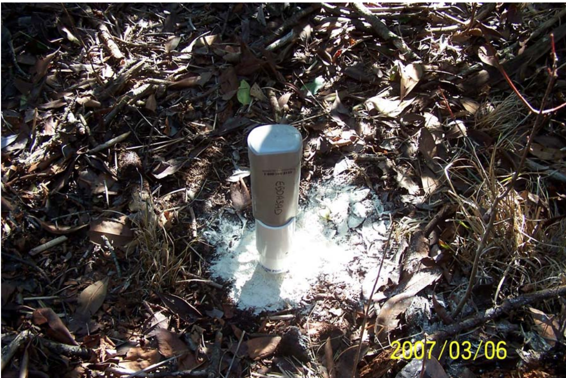
Typical well installation in reference area.
