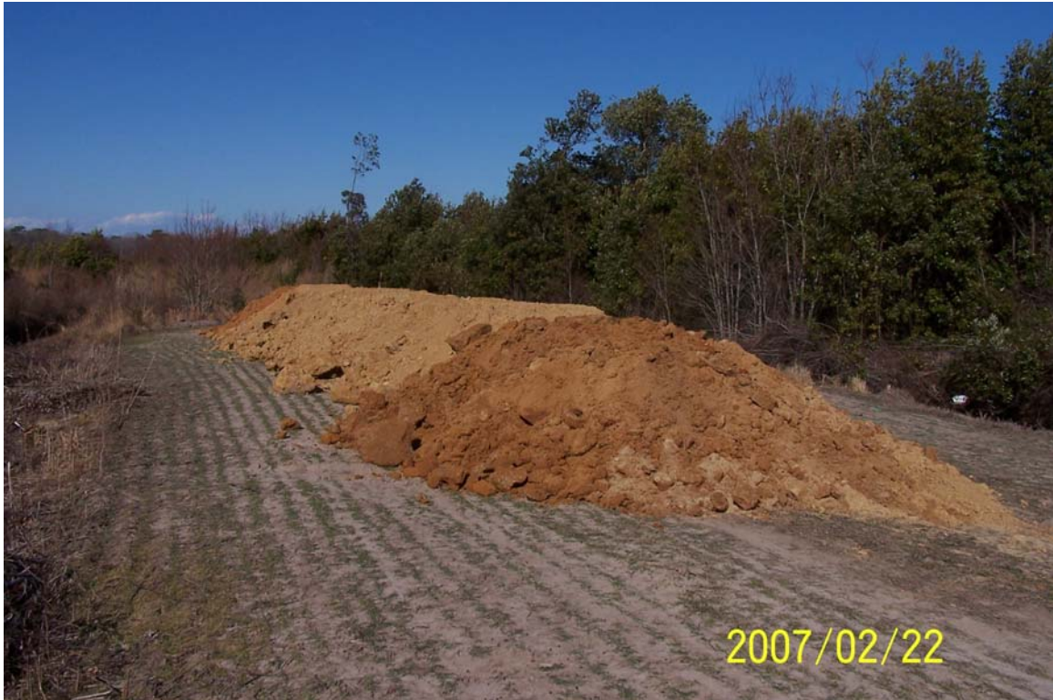
Clean fill material used for ditch plugs.
