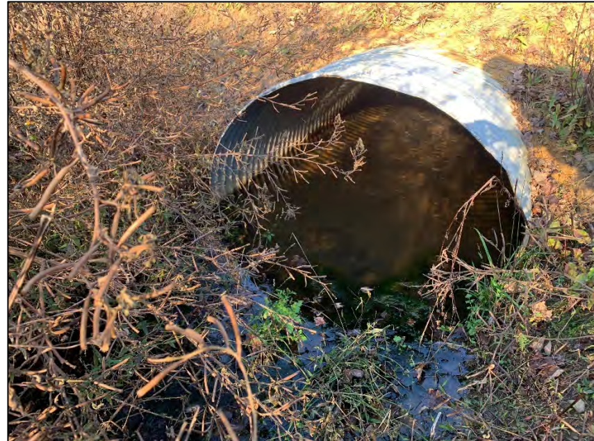
BB-C - Farm Culvert Exit - (11/8/2023)
