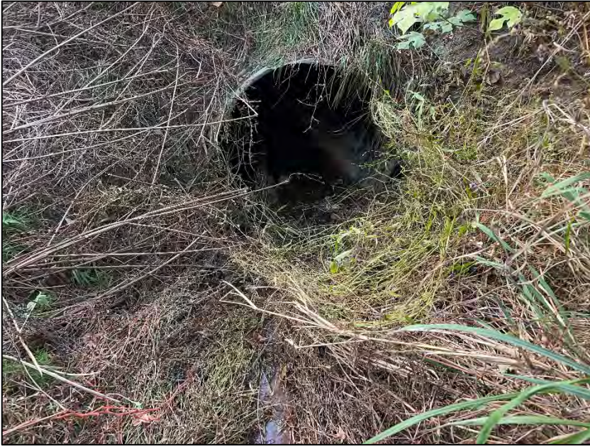
BB-B - E Darden Rd. Culvert Entrance - (11/7/2023)
