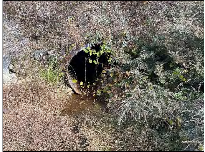
BB-C – E Darden Rd. Culvert Exit (11/7/2023)
