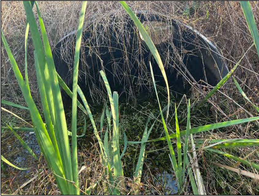
DE4-B – Farm Culvert Entrance - (11/8/2023)
