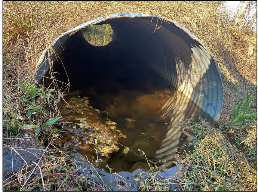
DE4-B – Farm Culvert Exit - (11/8/2023)
