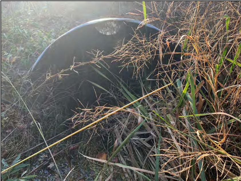
BB-C - Farm Culvert Entrance - (11/8/2023)
