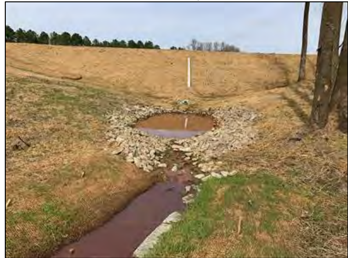
Siphon to stream (03/23/2023)
