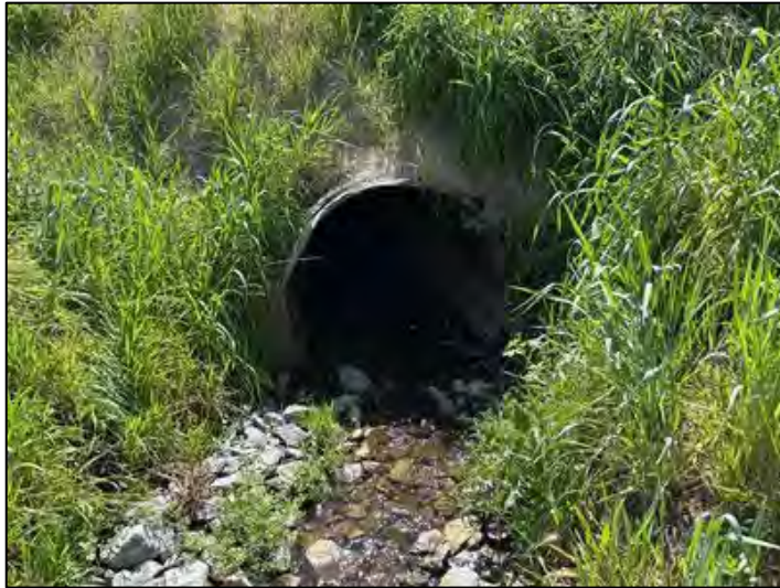
BB-B - E Darden Rd. Culvert Entrance - (03/23/2023)
