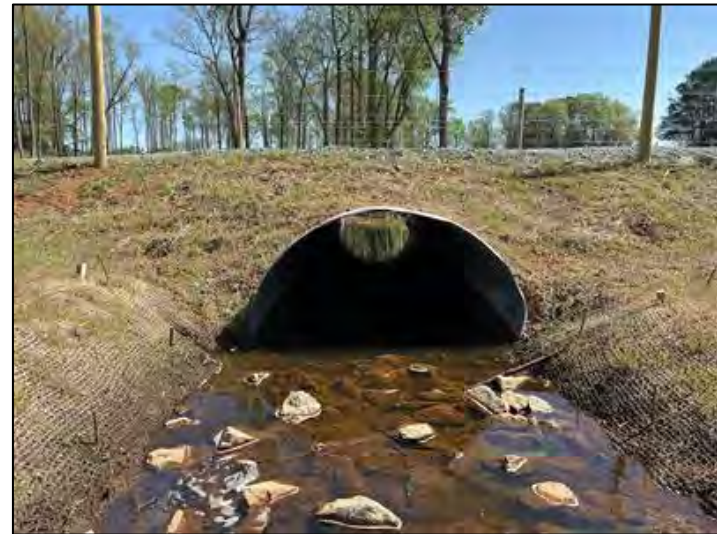
BB-C - Farm Culvert Exit - (03/30/2023)
