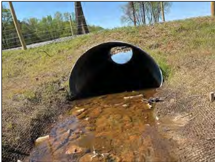
BB-C - Farm Culvert Entrance - (03/30/2023)
