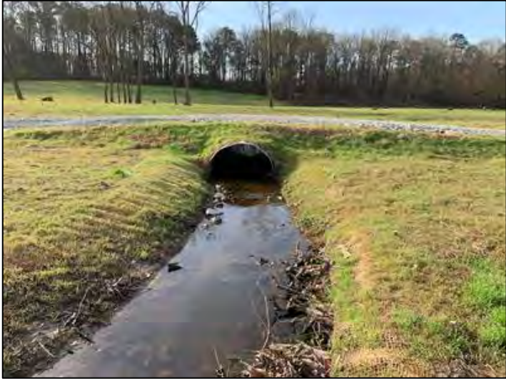
DE4-B – Farm Culvert Entrance - (03/1/2023)
