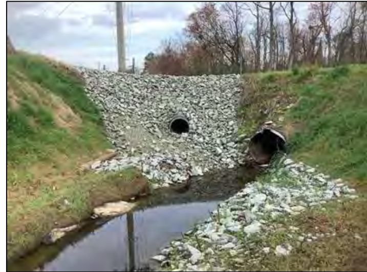
BB-C - E Darden Rd. Culvert Exit (03/30/2023)
