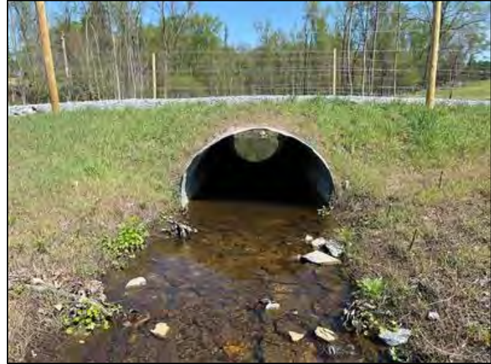
DE4-B – Farm Culvert Exit - (03/30/2023)
