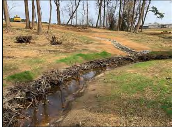
Brush toe and spillway (03/01/2023)
