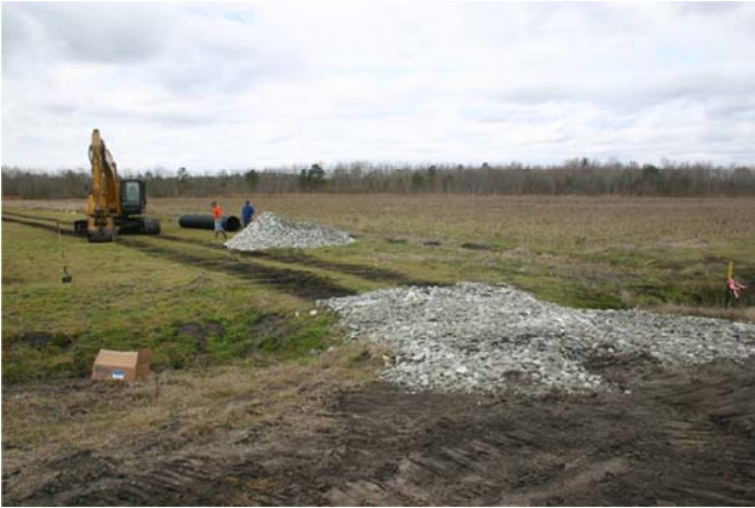
Construction Staging Area
