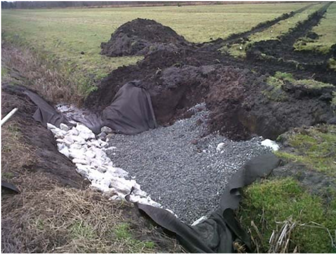
Pipe Outlet, Rip-Rap Headwall
