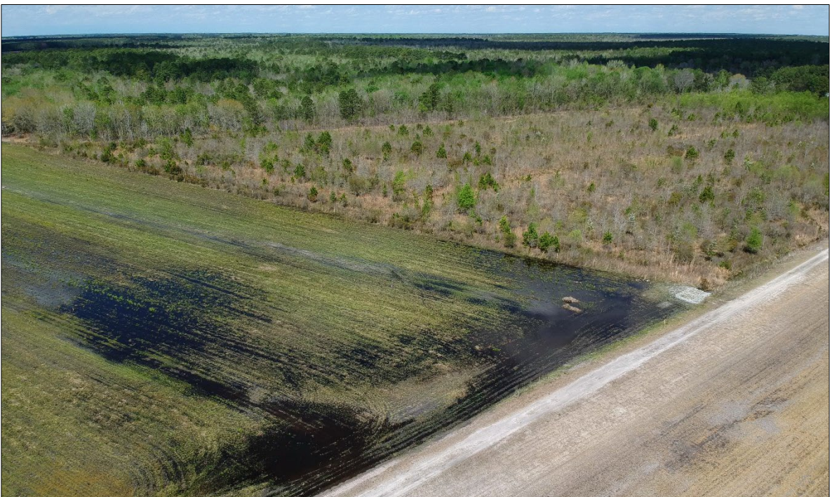
Photo 02: Looking northwest at Project's eastern outfall – boundary with Sliver Moon Site
