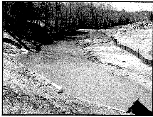
Photo 14 – AR2 downstream of box culverts
