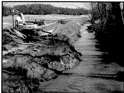
Photo 12 – Upstream of golf cart crossing AR1 and golf course under construction
