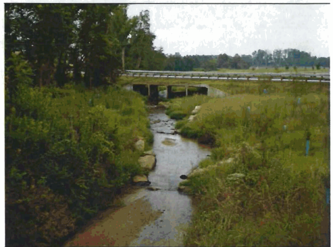
APP14 - AR1 STA 23+19 from Golf Cart Bridge
