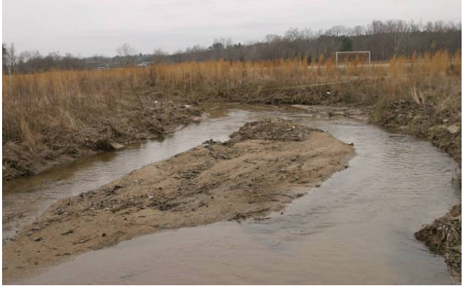
Photo of Cross-Section AR3-3 - Looking Downstream @ STA 38+15
