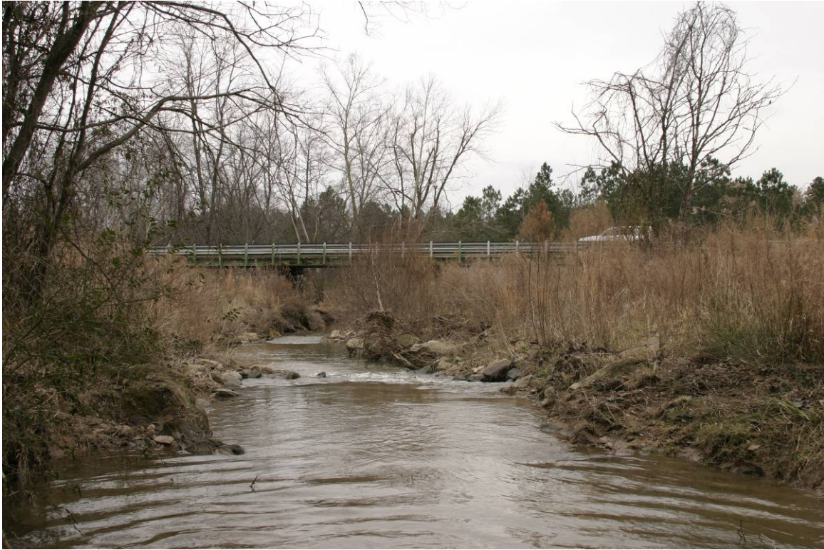
SPP83 SR3 STA 52+00 PROJECT END_JFR
