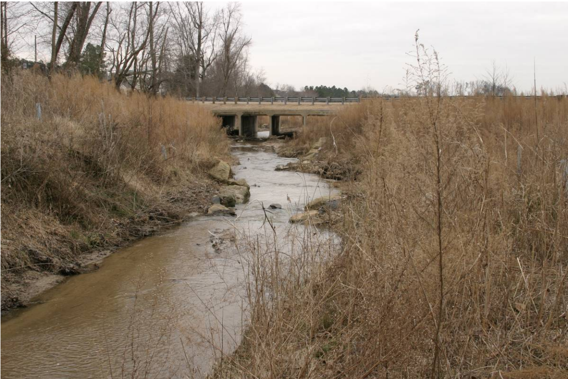
APP14 AR1 STA 23+19 FROM GOLF CART BRIDGE
