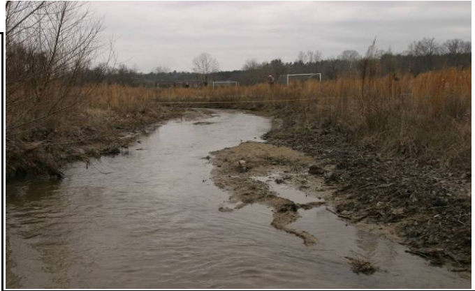
Photo of Cross-Section AR3-4 - Looking Downstream @ STA 41+00
