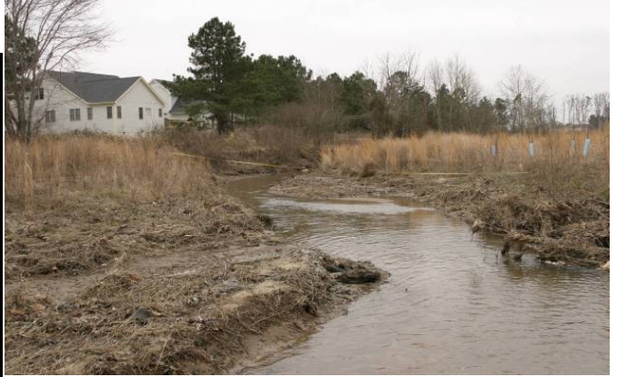
Photo of Cross-Section AR3-2 - Looking Downstream @ STA 35+15
