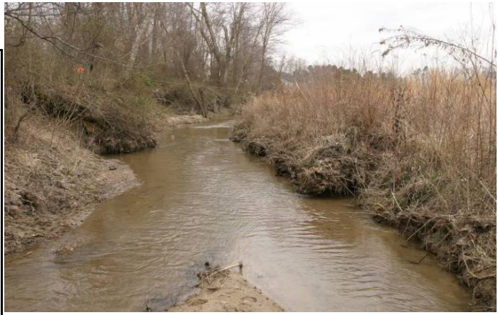
Photo of Cross-Section AR2-1 - Looking Downstream @ STA 27+90
