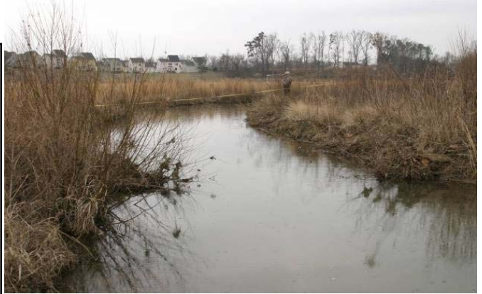
Photo of Cross-Section SR2-4 - Looking Downstream @ STA 32+45
