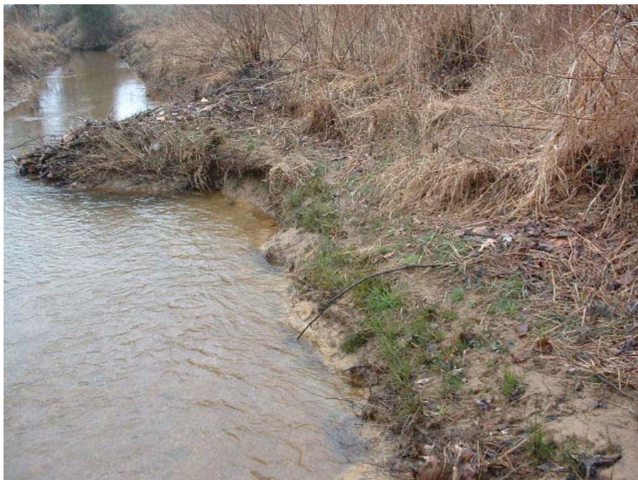
VPA 14. Smith Creek Station 26+50. Previous bare bank behind beaver dam removed. Now a hardy stand of Juncus sp. is establishing. Not a problem location.
