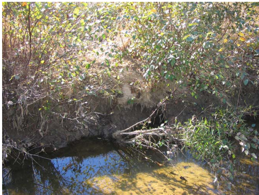
VPA2. Smith Creek Station 40+40. Un-vegetated Bank
