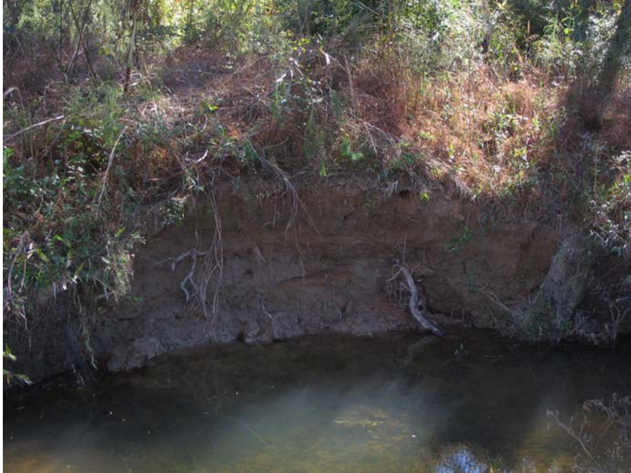
VPA13. Austin Creek Station 34+00. Bare bank.
