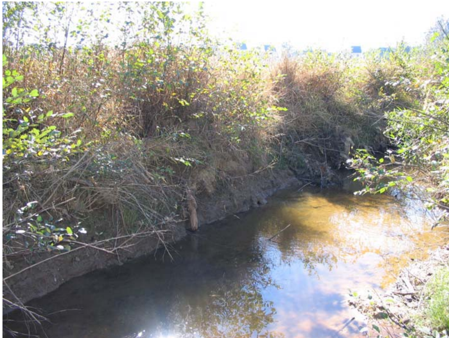
VPA4. Smith Creek Station 36+60. Un-vegetated Bank
