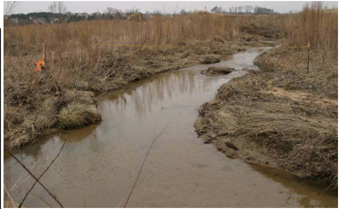
Photo of Cross-Section SR1-3 - Looking Downstream @ STA 11+30
