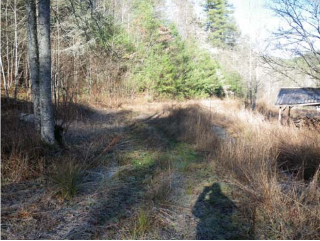
VPA1 – Easement encroachment/buffer impact from access road paralleling the upstream limits of UT3-Reach 2 (looking downstream from left floodplain)
