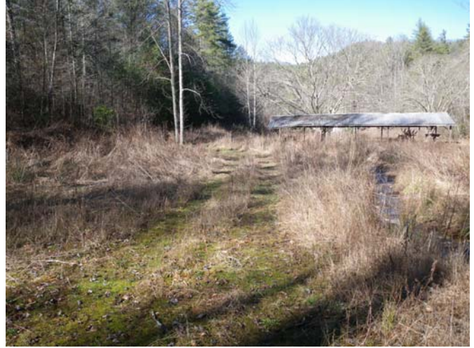
VPA1 – Easement encroachment/buffer impact from access road paralleling the upstream limits of UT3-Reach 2 (looking downstream from left floodplain)
