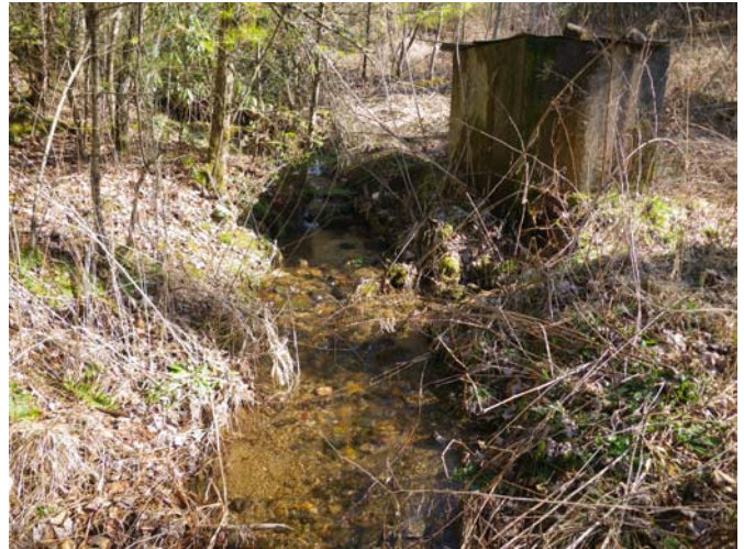
Photo Point 1: looking upstream (out of easement)
