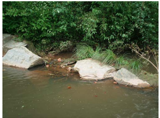
PA14 facing left bank (9/10/08)
