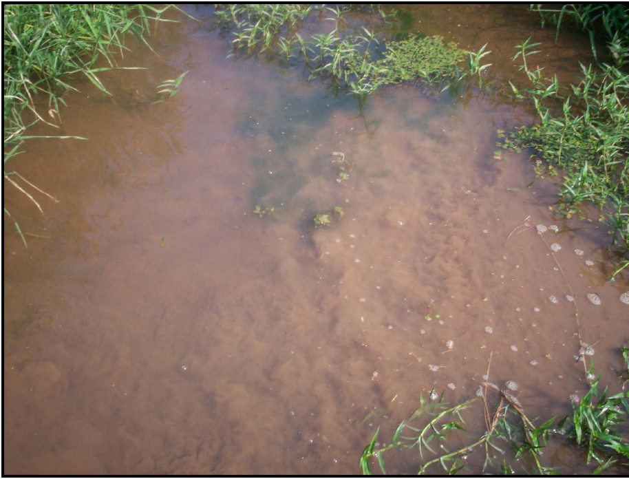
SPA 7. Buried log vane in UT1A North at STA 50+00.
