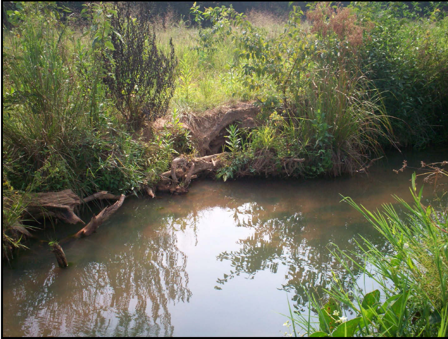
SPA 9. Minor erosion at root wad in UT1A North at STA 60+00.
