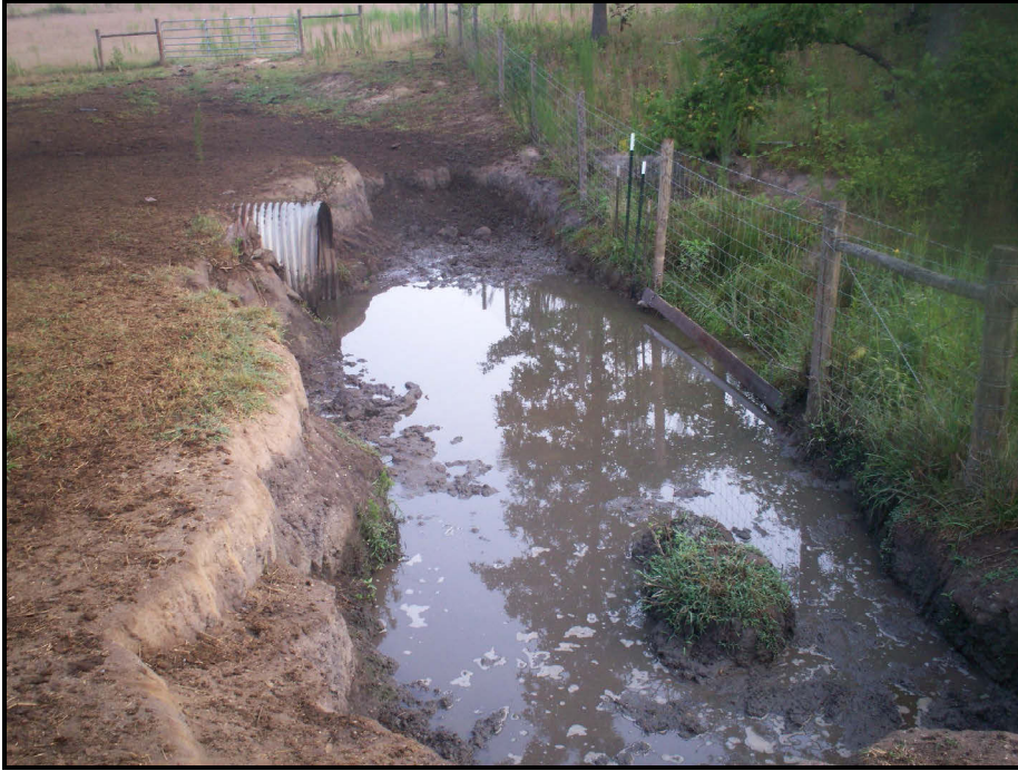
Upstream of culvert at cattle crossing in UT5 South.
