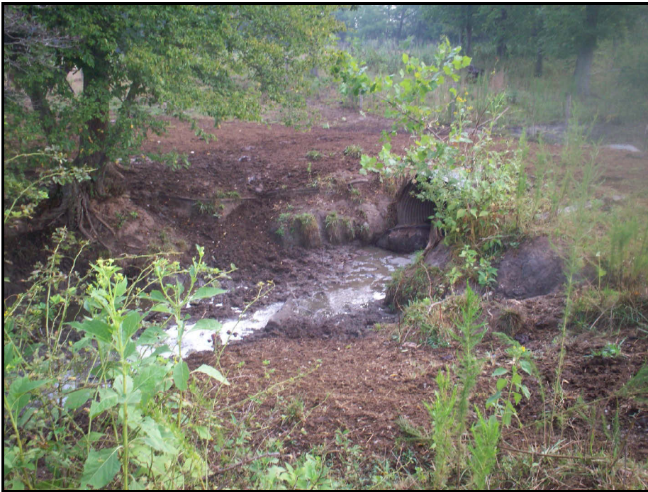
Downstream of culvert at cattle crossing in UT5 South.
