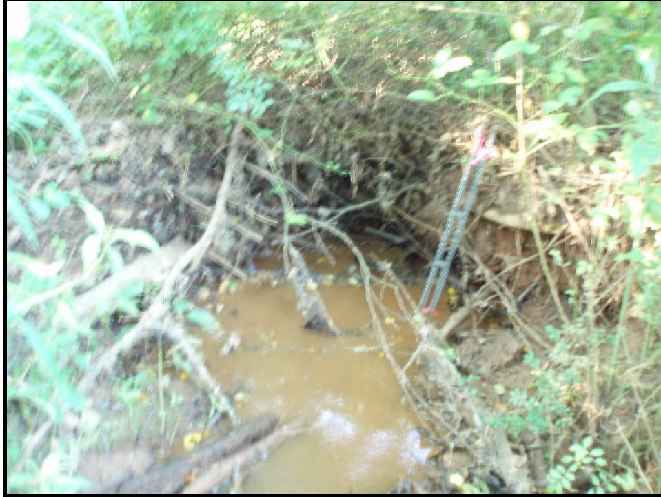
UT1A station 33+00. Debris jam and right bank erosion.
