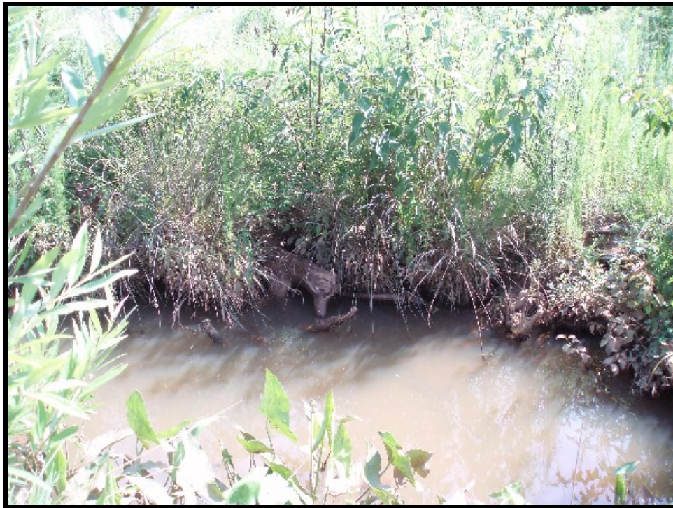
UT1B station 60+00. Unstable root wad.
