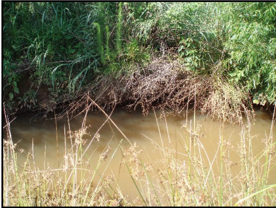
UT1B station 58+40. Unstable root wad.
