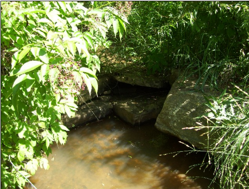
M2 STA 28+70 Perched header on rock cross vane
