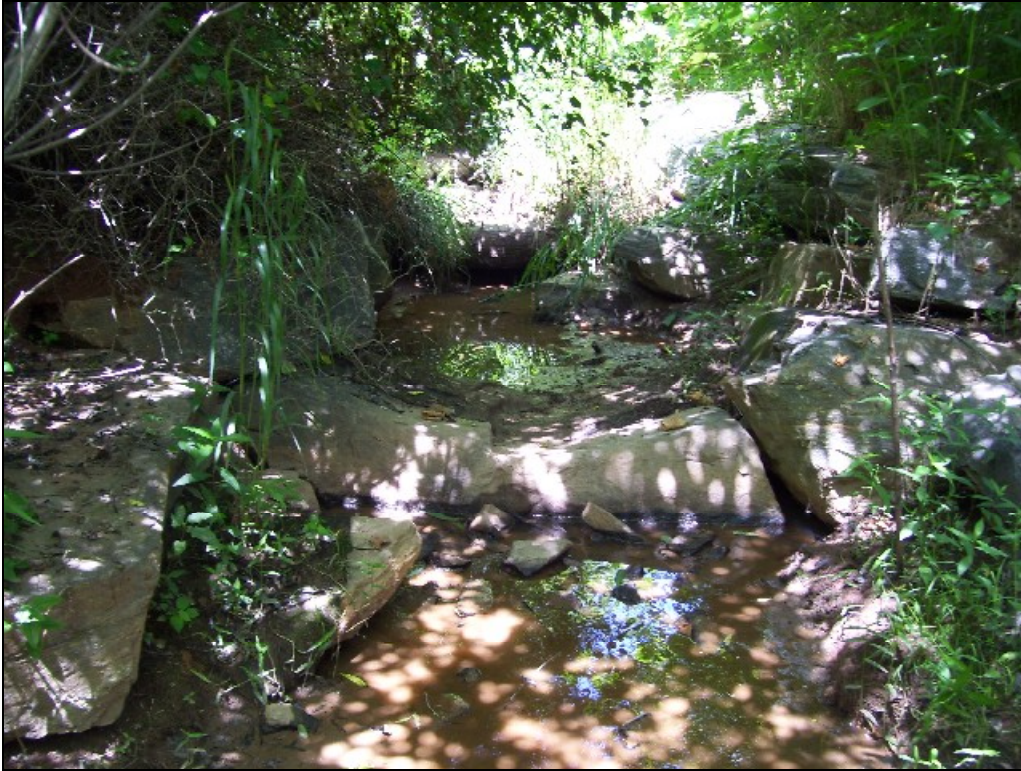
UT4 STA 18+60 Piping beneath lower header rocks of step pool system
