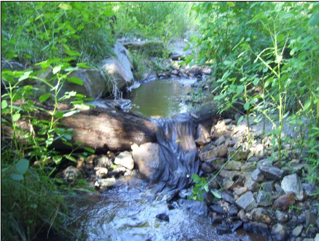
M2 STA 38+10 Lower header rocks perched in step pool system
