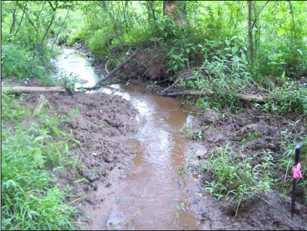
UT1A STA 10+00–35+00 Typical minor bank erosion from cattle access
