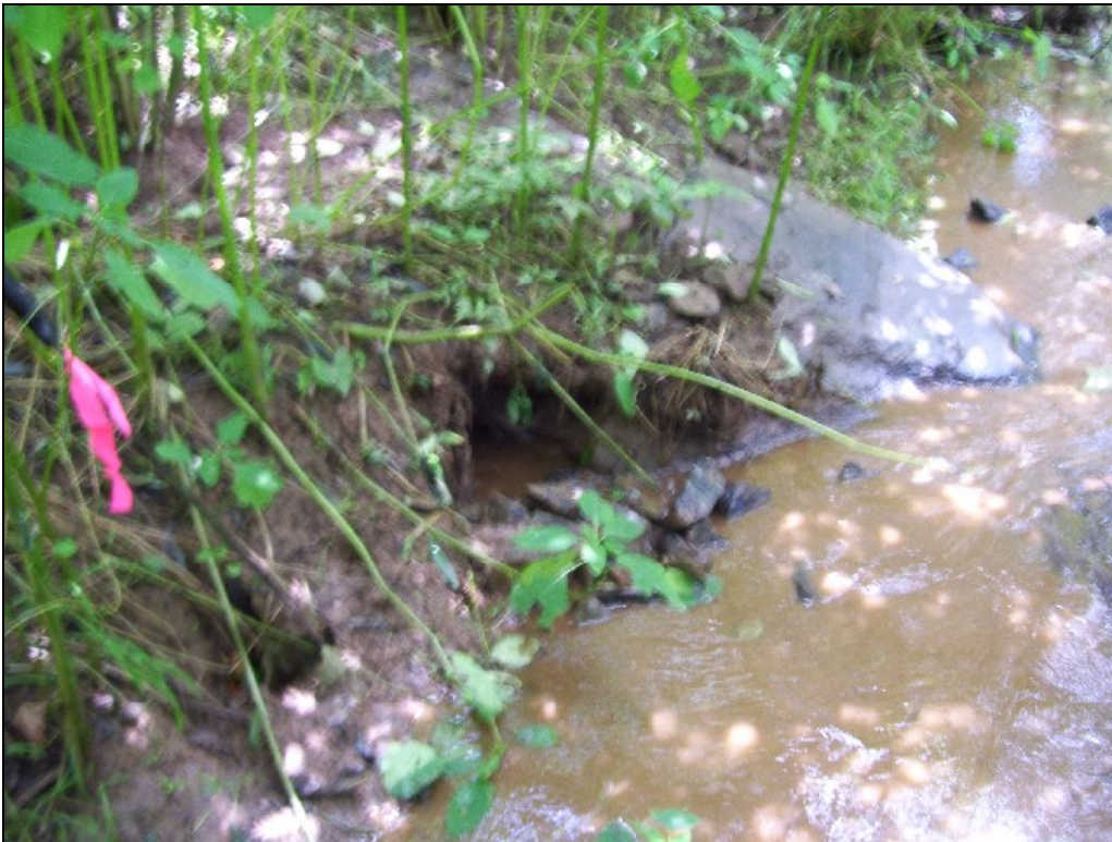
UT2A STA 21+50 minor piping around header rock on left bank of constructed riffle
