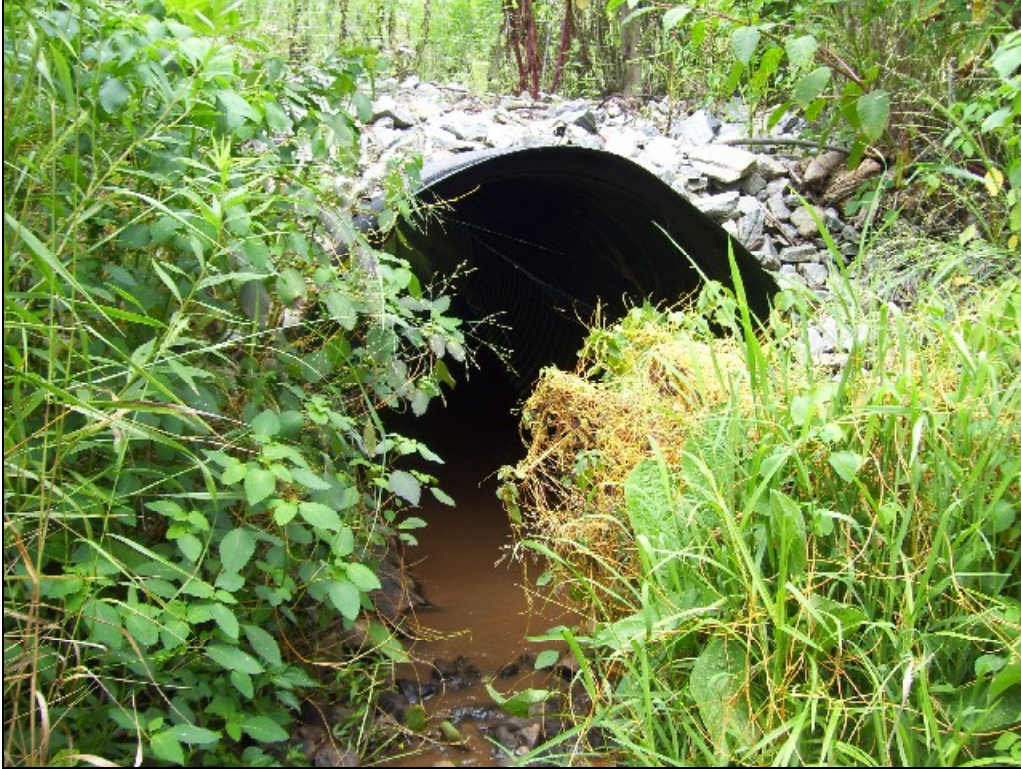
Typical stable culvert outlet
