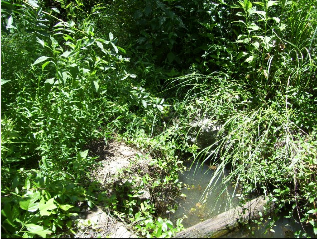
UT5 STA 24+50 Piping below header rock of rock cross vane
