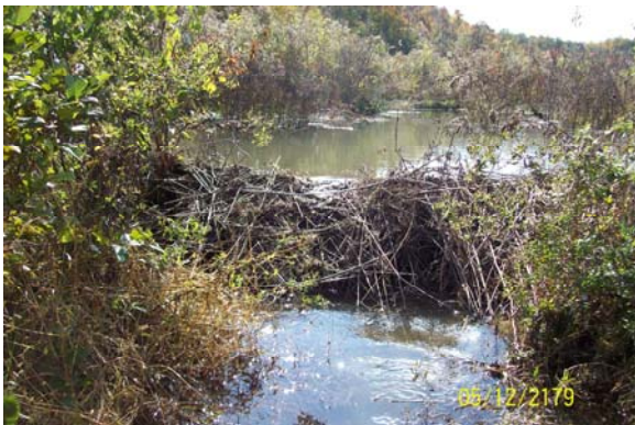
Beaver dam at Station 176+50
