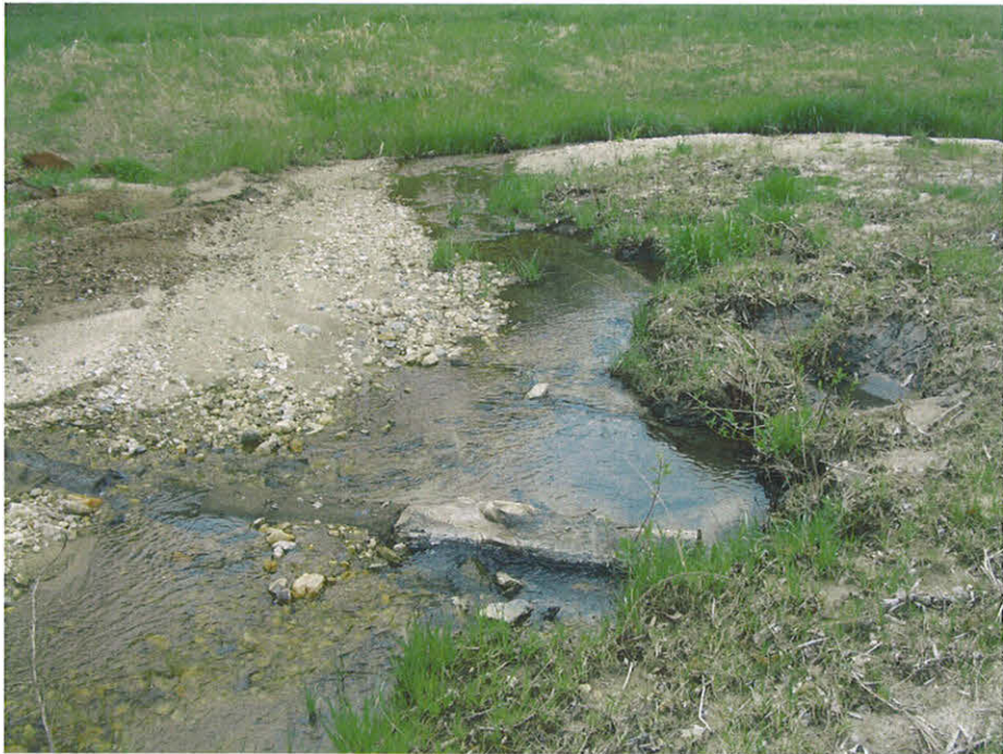
SPA 4 Bank scour along Tributary B at station 19+70. (EMH&T, Inc. 4/14/07)
