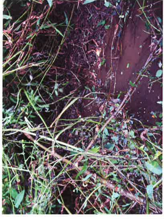
Cross-section photo – looking downstream Channel completely obscured by vegetation.
