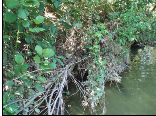
Spring Valley 2006 - Problem Area 8
