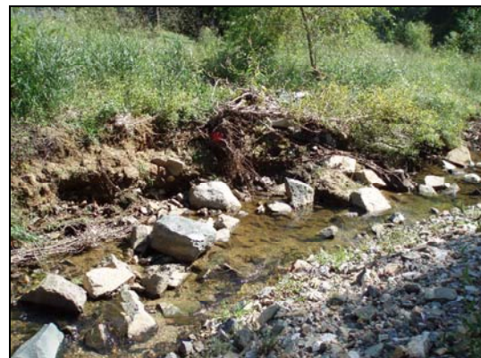
Spring Valley 2006 - Problem Area 6
