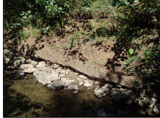
Spring Valley 2006 - Problem Area 2
