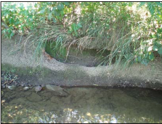
Spring Valley 2006 - Problem Area 9
