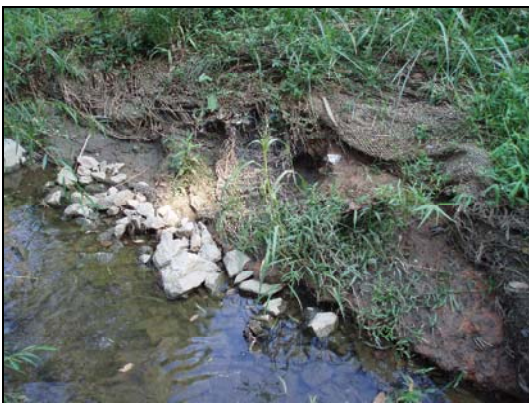
Spring Valley 2006 - Problem Area 11
