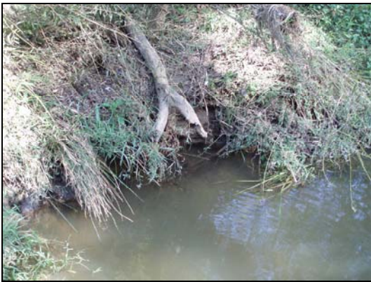
Spring Valley 2006 - Problem Area 15
