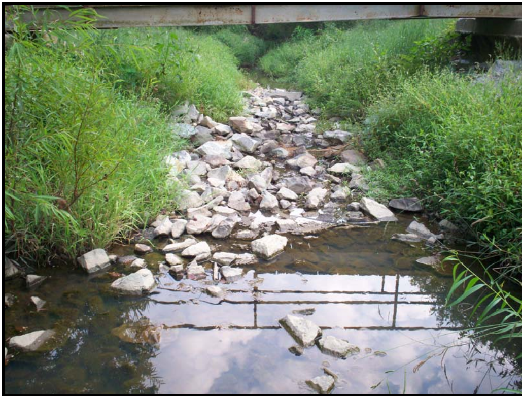
Photo Point #5 - Station 21+00 Downstream
