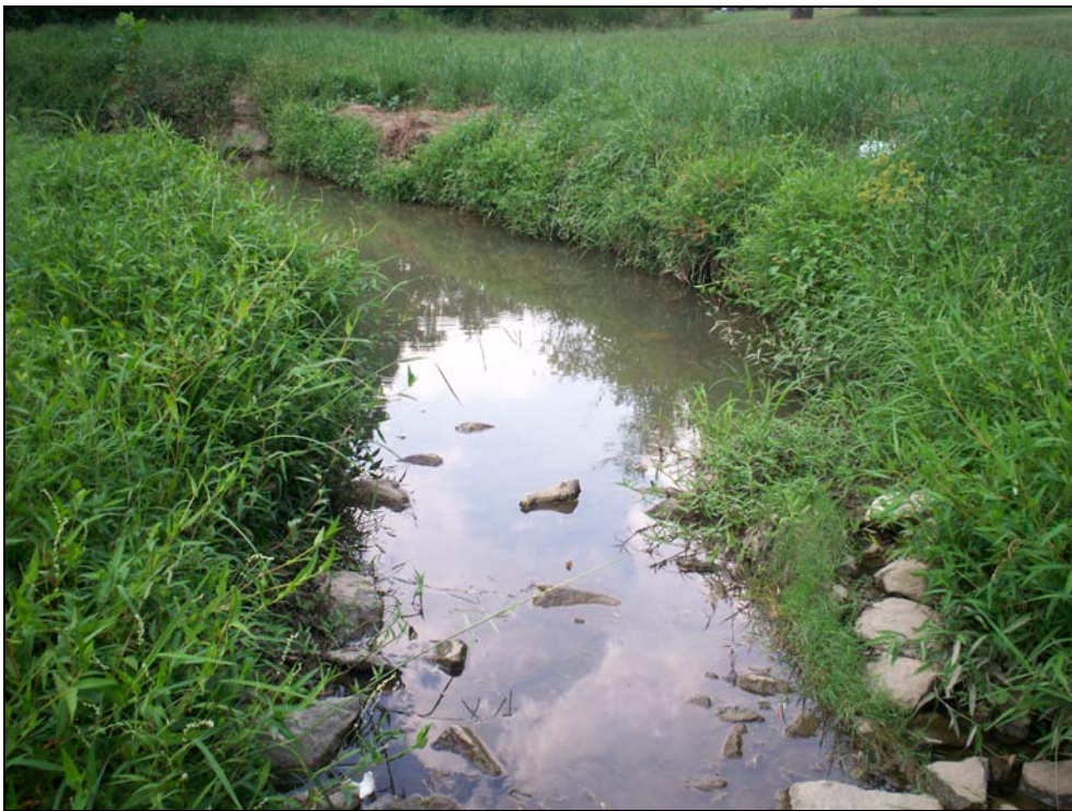
Problem Area # 18. Lower portion of project lacks of woody vegetated buffer. Station 21+00 Upstream.
