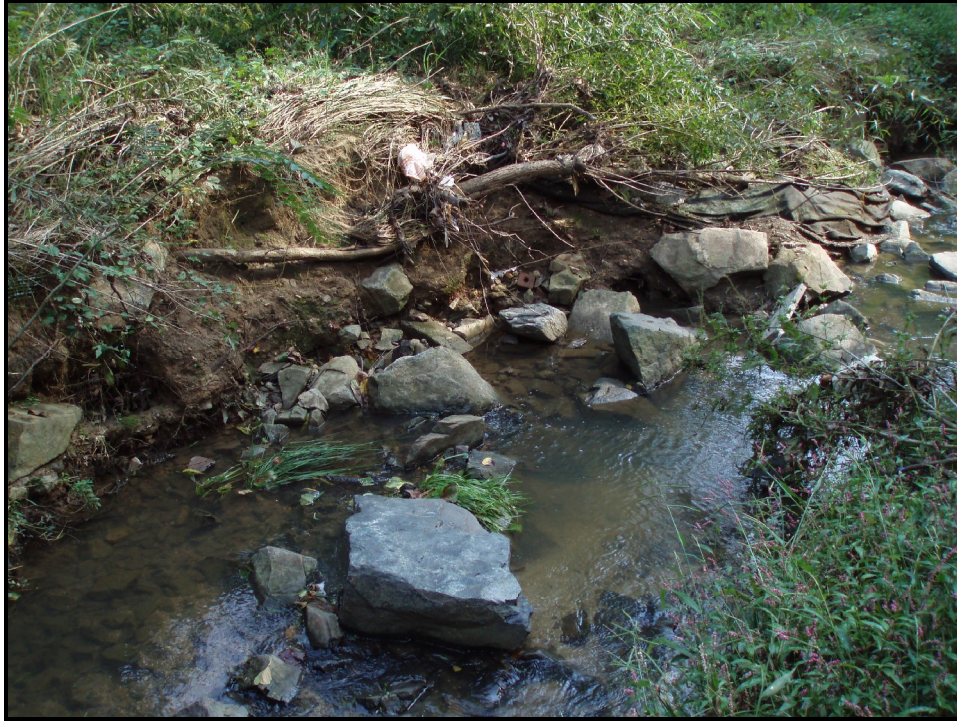
PA #3 – Left bank erosion; lack of rooted vegetation. Sta. 16+50
