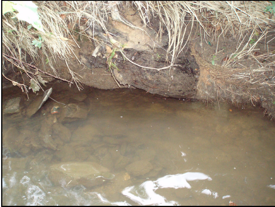
PA #7 – Left bank erosion/undercut; lack of rooted vegetation. Sta. 18+80
