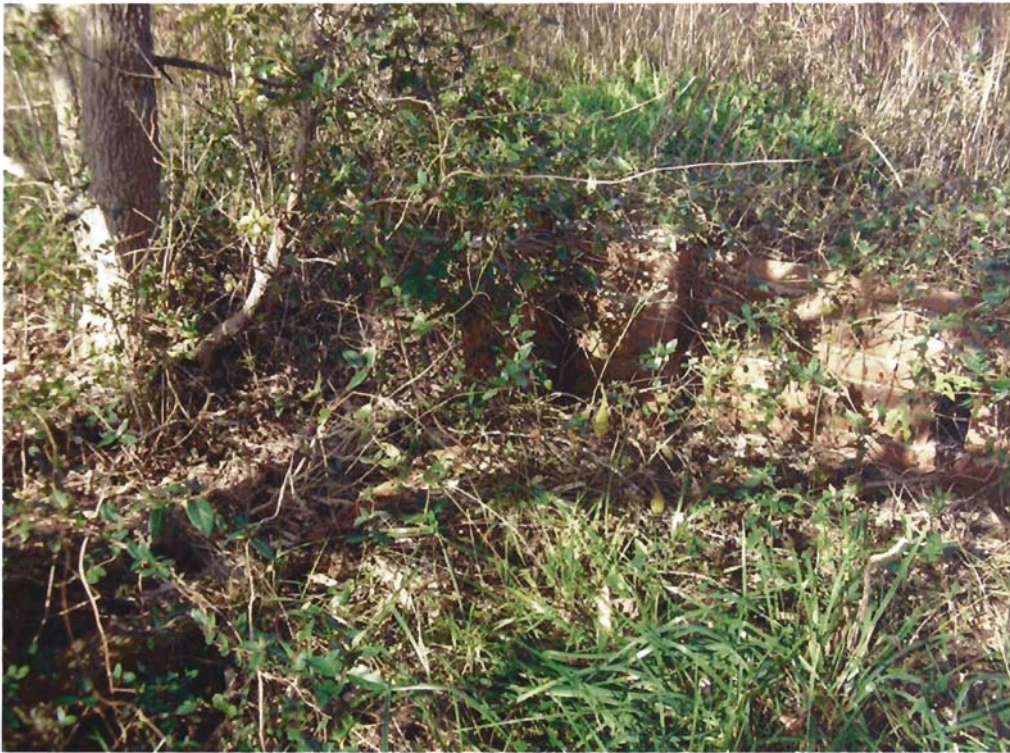
Photo 4: Brick foundation covered in vines
