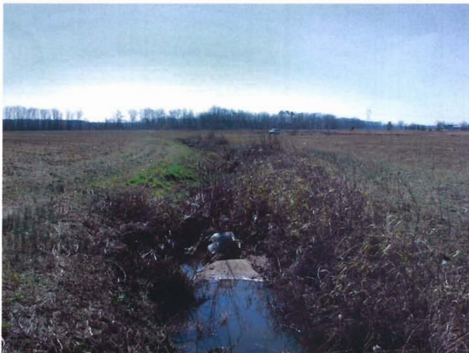
Channel upstream of Reach B, north of Webb Farm Rd.
