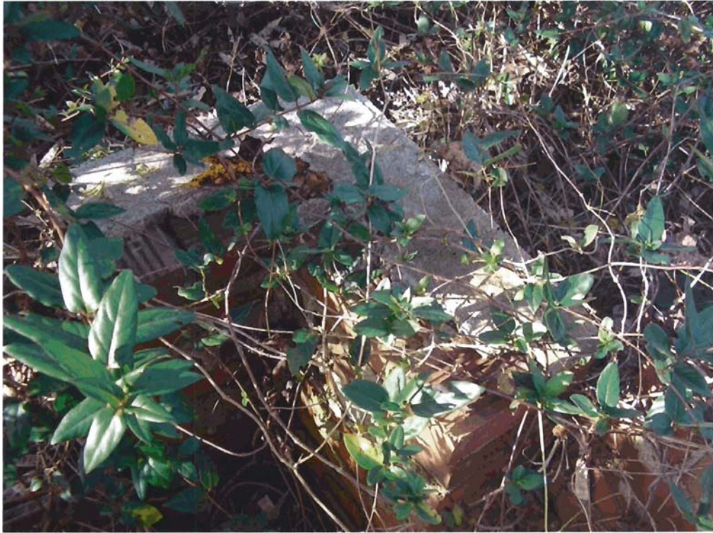
Photo 3: Close up of brick foundation
