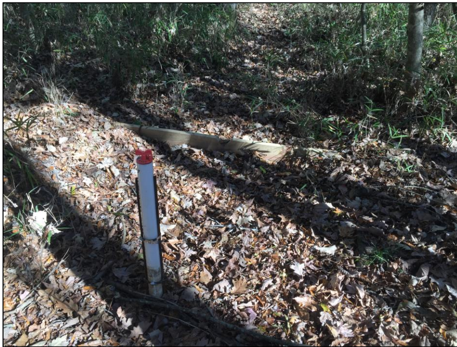
Photo 2. Weir at Gauge 3
