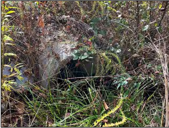
Photo Point 23C – UT2, Sta. 10+47 Upstream Invert (10/26/2023)
