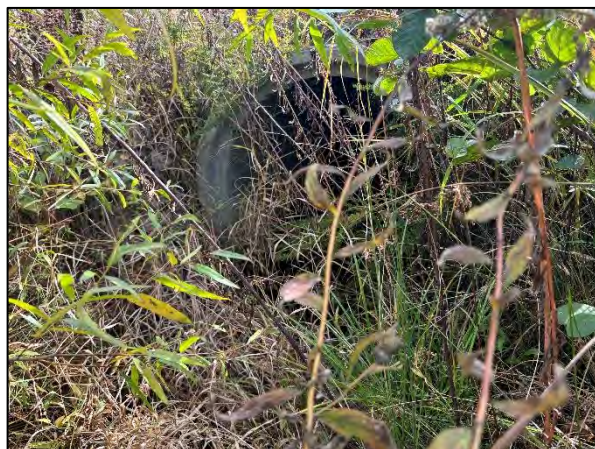
Photo Point 33C – UT3 Reach 2, Sta. 27+44 Upstream Invert (10/26/2023)
