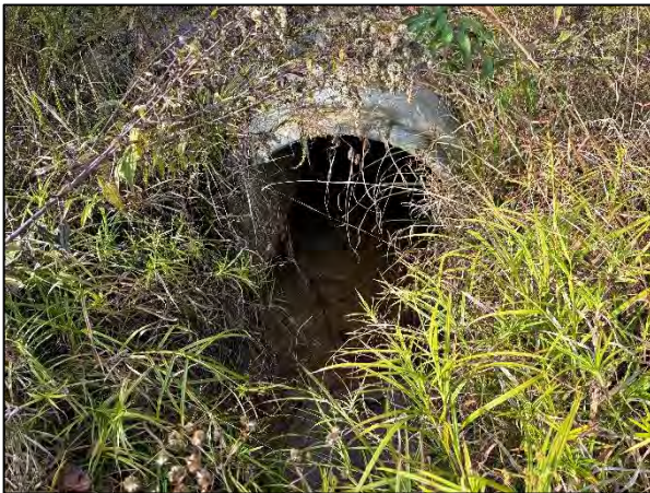
Photo Point 27D – UT3 Reach 1, Sta. 11+51 Downstream Invert (10/26/2023)
