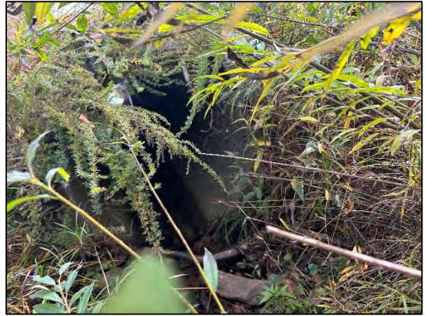
Photo Point 27C – UT3 Reach 1, Sta. 11+51 Upstream Invert (10/26/2023)
