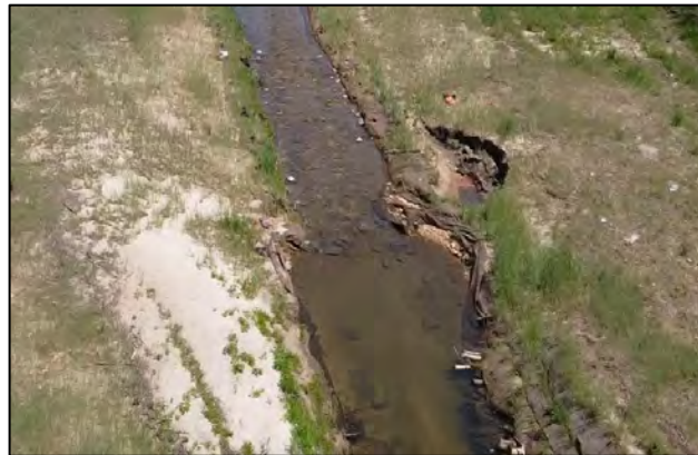
CPA-1, upstream section, facing downstream (5/10/2023)
