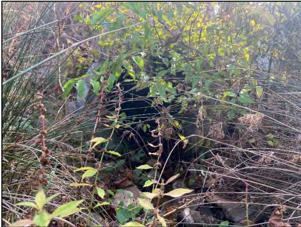
Photo Point 14C – UT1, Sta. 12+91 Upstream Invert (10/26/2023)
