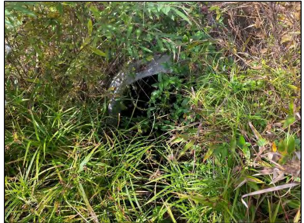
Photo Point 14D – UT1, Sta. 12+91 Downstream Invert (10/26/2023)
