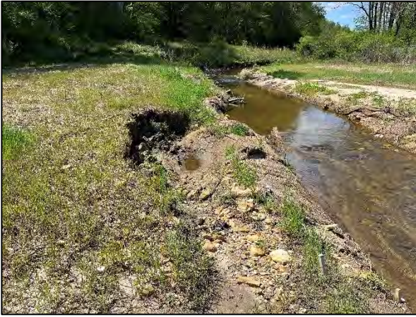
CPA-1, upstream section, facing upstream (4/20/2023)
