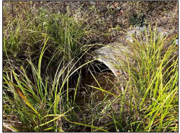
Photo Point 23D – UT2, Sta. 10+47 Downstream Invert (10/26/2023)
