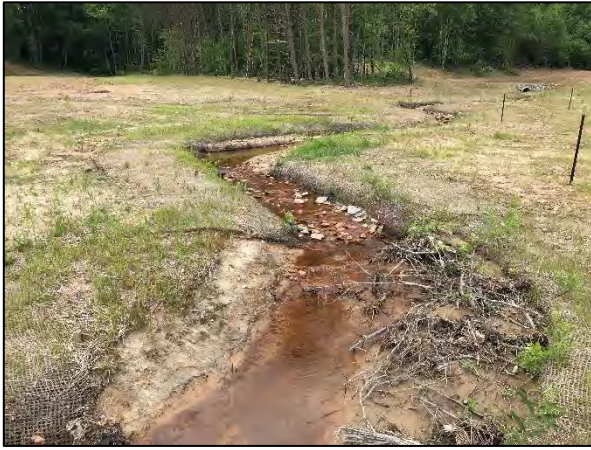
Photo Point 15 – UT1, Sta. 15+52 Facing Upstream (6/11/2020)
