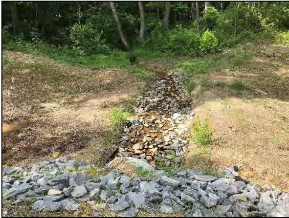
Photo Point 23A – UT2, Sta. 10+47 Facing Upstream (6/11/2020)
