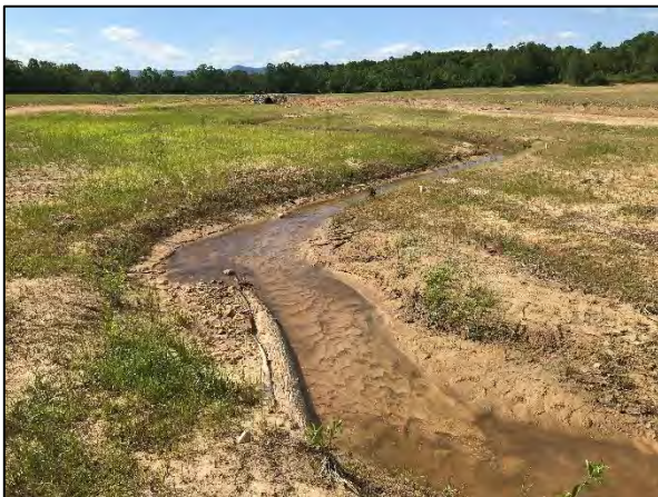
Photo Point 34 – UT3 Reach 2, Sta. 30+47 Facing Upstream (6/11/2020)
