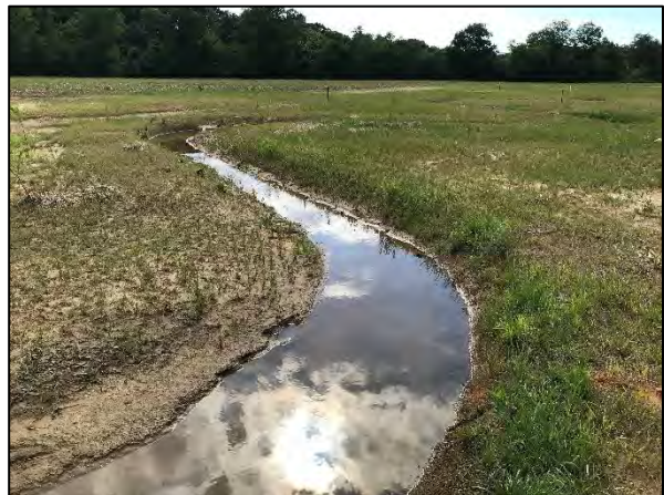
Photo Point 35 – UT3 Reach 2, Sta. 37+79 Facing Upstream (6/11/2020)
