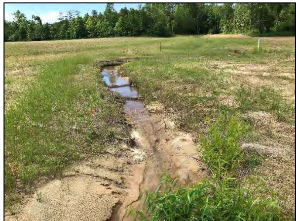
Photo Point 30 – UT3 Reach 1, Sta. 18+28 Facing Upstream (6/11/2020)
