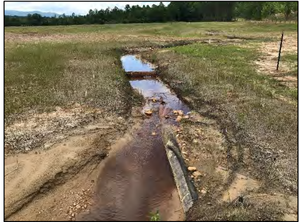
Photo Point 18 – UT1, Sta. 22+81 Facing Upstream (6/11/2020)
