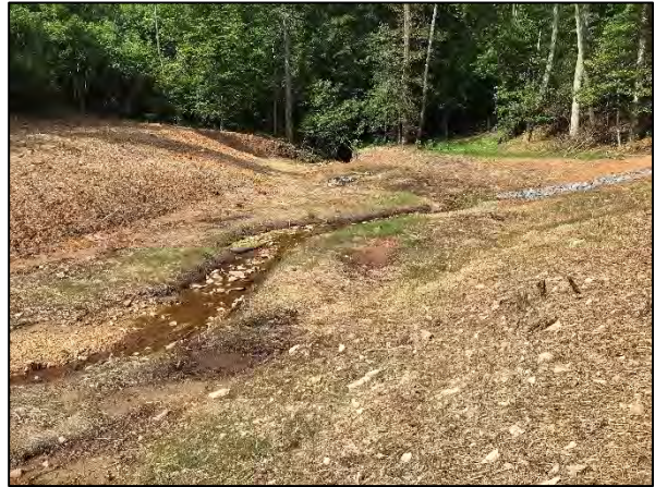
Photo Point 13 – UT1, Sta. 10+84 Facing Upstream (6/11/2020)
