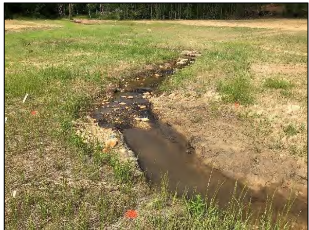
Photo Point 25 – UT2, Sta. 14+65 Facing Upstream (6/11/2020)
