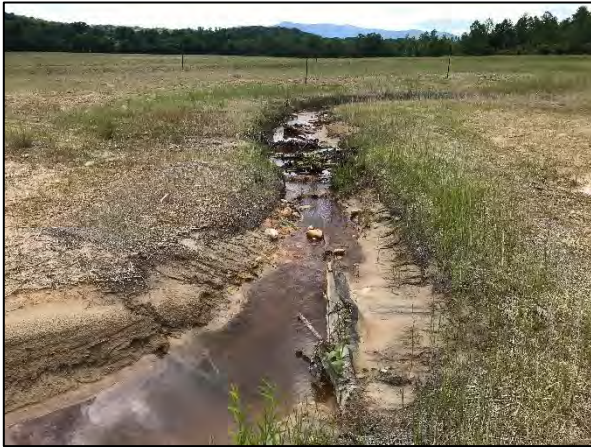
Photo Point 17 – UT1, Sta. 21+12 Facing Upstream (6/11/2020)
