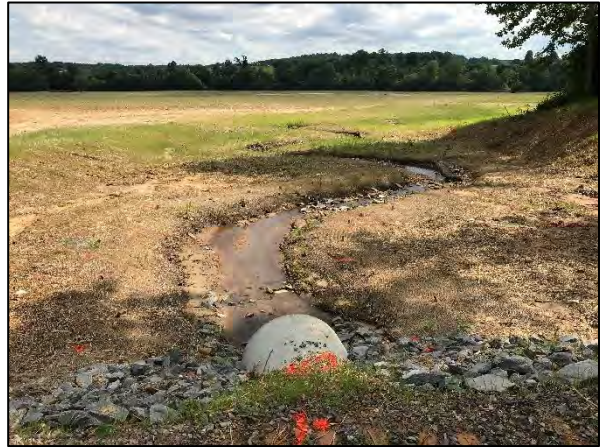
Photo Point 23B – UT2, Sta. 10+47 Facing Downstream (6/11/2020)
