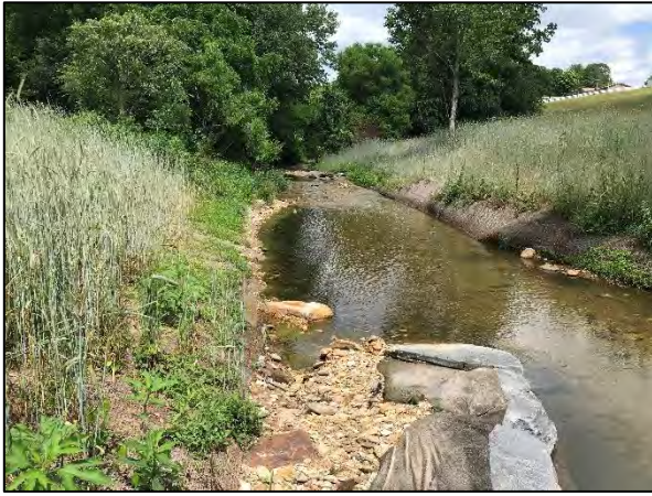
Photo Point 1A – Moores Fork Reach 1, Sta. 11+81 Facing Upstream (6/11/2020)
