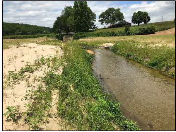
Photo Point 12A – Moores Fork Reach 3, Sta. 50+54 Facing Upstream (6/11/2020)
