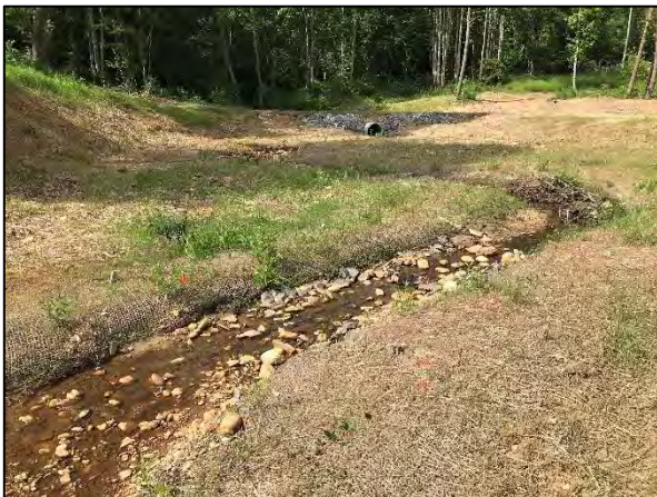
Photo Point 24 – UT2, Sta. 11+57 Facing Upstream (6/11/2020)
