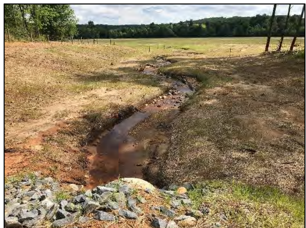
Photo Point 14B – UT1, Sta. 12+91 Facing Downstream (6/11/2020)
