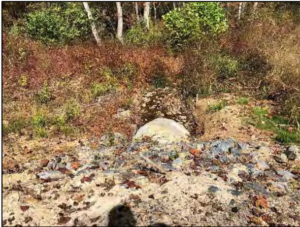
Photo Point 23A – UT2, Sta. 10+47 Facing Upstream (10/22/2020)
