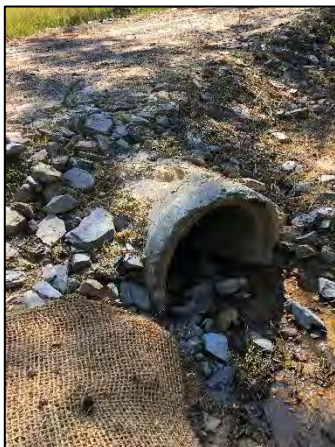
UT2 Culvert Opening Facing Upstream (09/22/2020)
