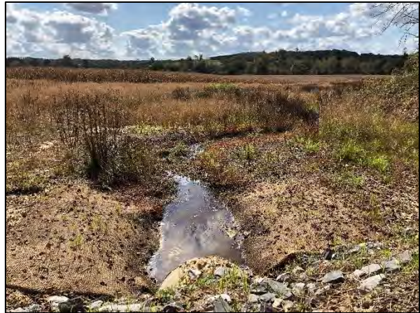
Photo Point 23B – UT2, Sta. 10+47 Facing Downstream (10/22/2020)
