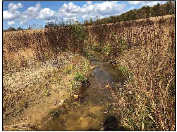
Photo Point 32 – UT3 Reach 2, Sta. 21+27 Facing Upstream (10/22/2020)
