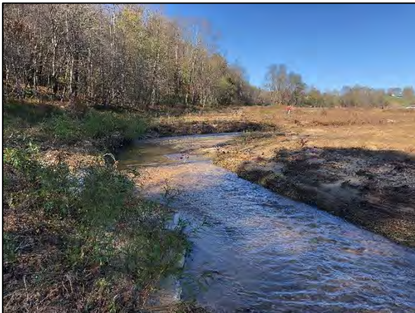
Photo Point 8 – Moores Fork Reach 2, Sta. 33+48 Facing Upstream (11/3/2020)
