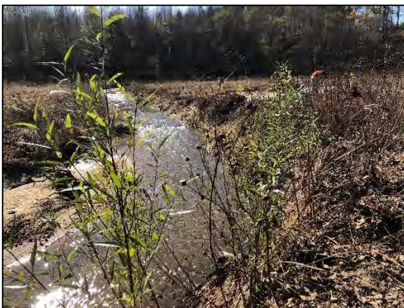
Photo Point 10 – Moores Fork Reach 2, Sta. 41+77 Facing Upstream (11/3/2020)
