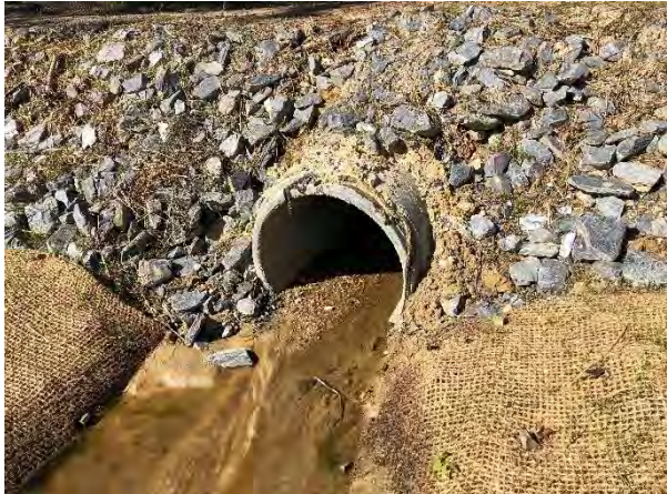
UT1 Culvert Opening Facing Upstream (09/22/2020)
