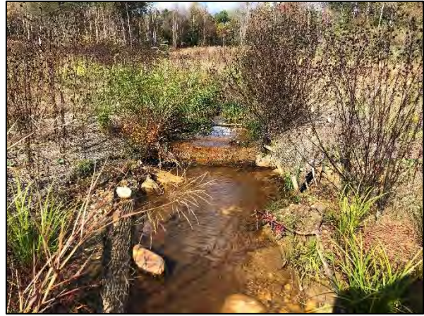
Photo Point 16 – UT1, Sta. 18+34 Facing Upstream (10/22/2020)
