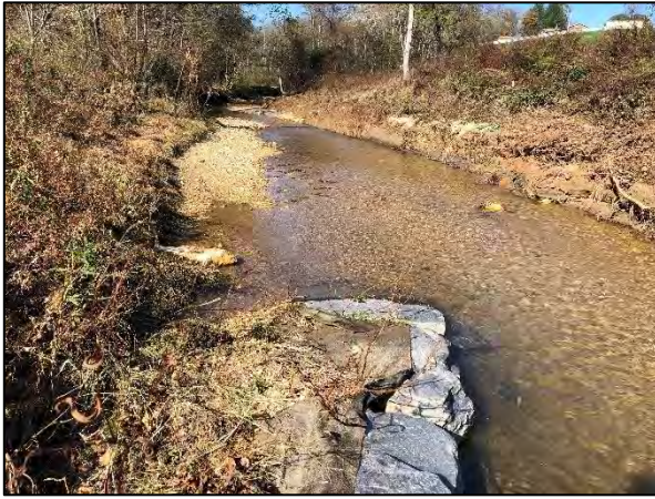
Photo Point 1A – Moores Fork Reach 1, Sta. 11+81 Facing Upstream (11/3/2020)
