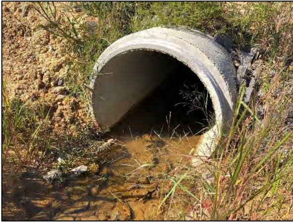
UT3 Reach 2 Culvert Opening Facing Upstream (09/22/2020)
