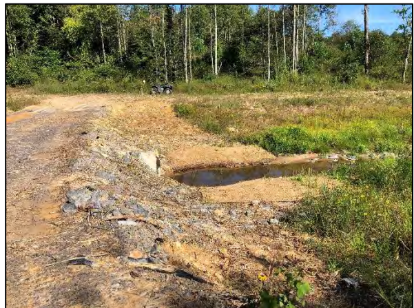
UT3 Reach 1 Culvert Opening Facing Culvert Downstream (09/22/2020)
