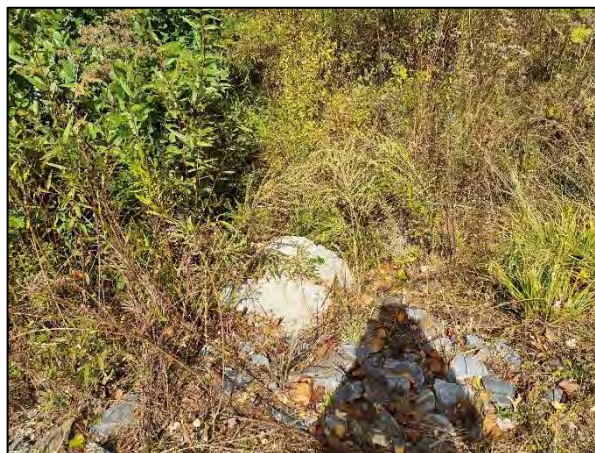
Photo Point 23A – UT2, Sta. 10+47 Facing Upstream (10/18/2022)
