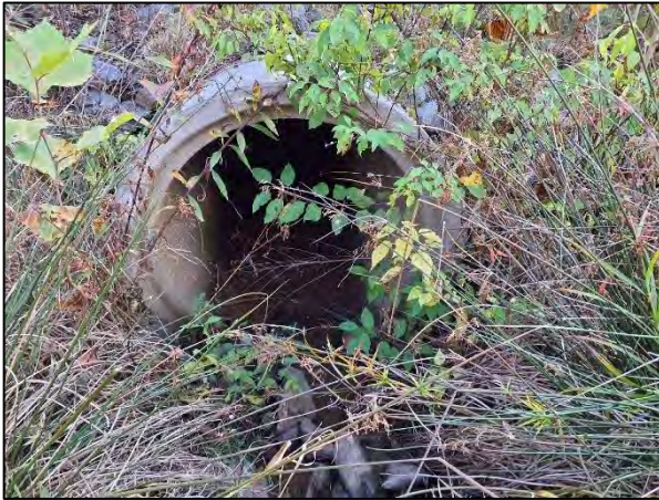
Photo Point 14C – UT1, Sta. 12+91 Upstream Invert (10/17/2022)
