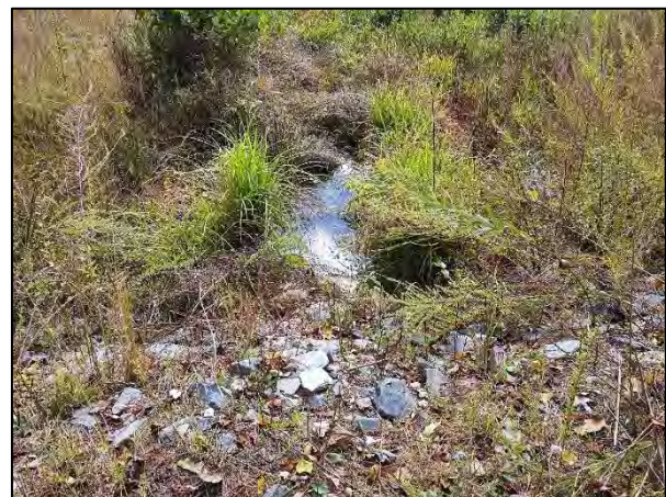
Photo Point 23B – UT2, Sta. 10+47 Facing Downstream (10/18/2022)
