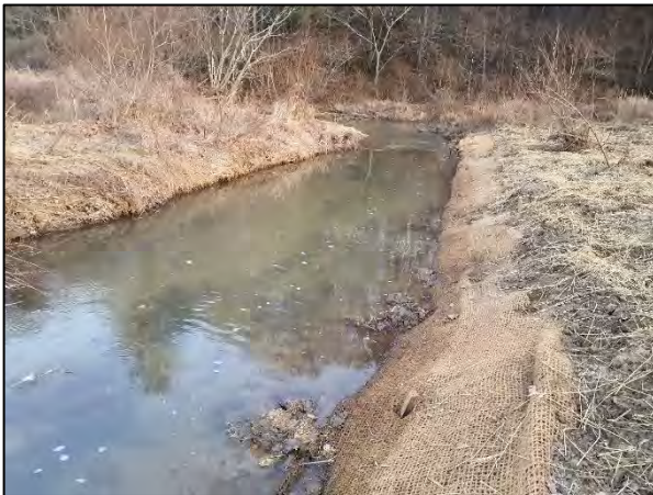
Photo Point 12B – Moores Fork Reach 3, Sta. 50+54 Facing Downstream (1/18/2023)
