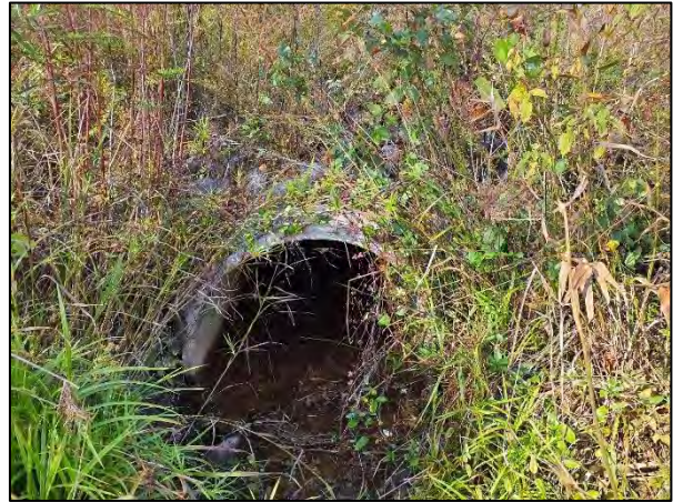
Photo Point 14D – UT1, Sta. 12+91 Downstream Invert (10/17/2022)
