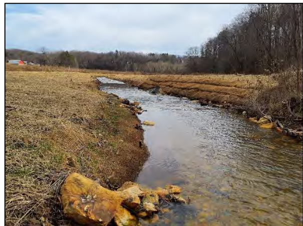
Photo Point 5 – Moores Fork Reach 2, Sta. 25+61 Facing Downstream (1/18/2023)
