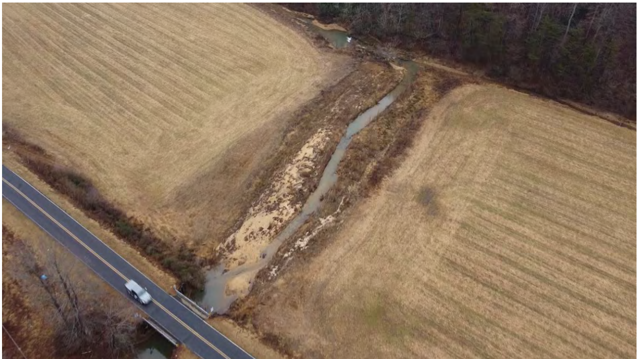
Site Overview – Moore's Fork Reach 3 (2/12/2022)
