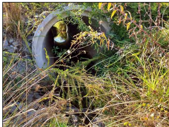
Photo Point 33C – UT3 Reach 2, Sta. 27+44 Upstream Invert (10/18/2022)
