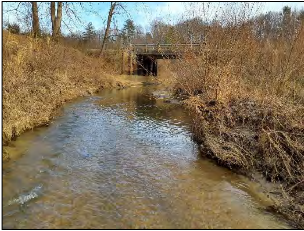
Photo Point 11B – Moores Fork Reach 2, Sta. 45+79 Facing Downstream (1/18/2023)
