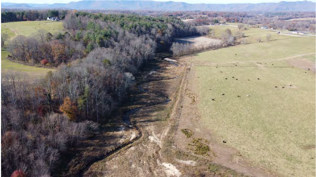
Site Overview – Moore's Fork Reach 2 (11/16/2021)
