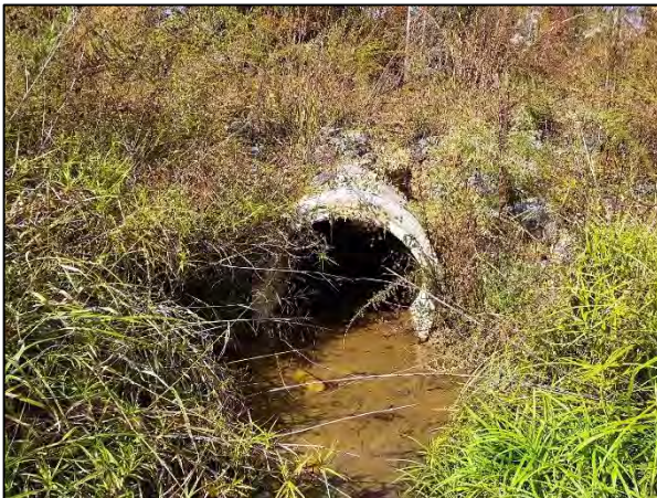
Photo Point 27D – UT3 Reach 1, Sta. 11+51 Downstream Invert (10/18/2022)
