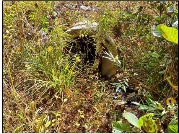
Photo Point 27C – UT3 Reach 1, Sta. 11+51 Upstream Invert (10/18/2022)
