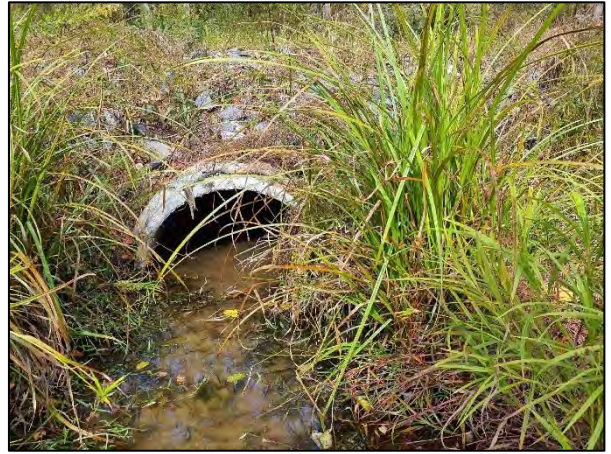
Photo Point 23D – UT2, Sta. 10+47 Downstream Invert (10/18/2022)
