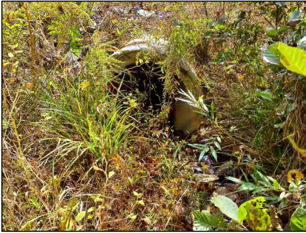
Photo Point 23C – UT2, Sta. 10+47 Upstream Invert (10/18/2022)
