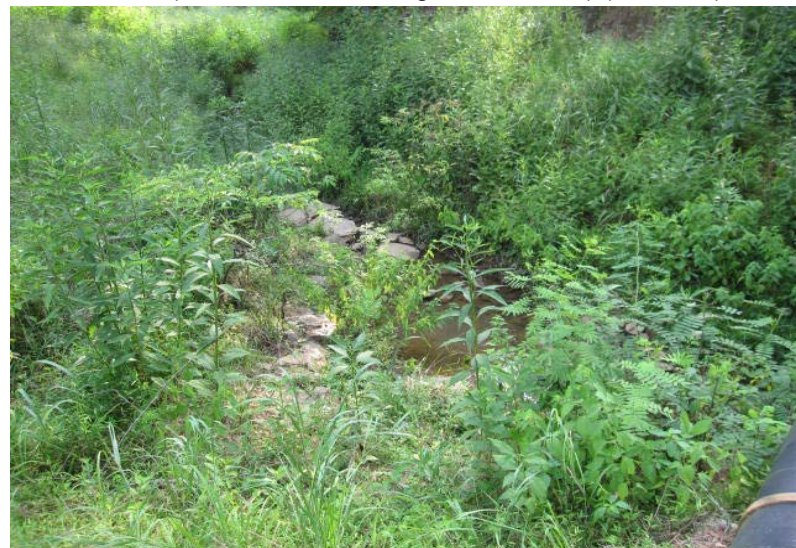
PP #10 (Sta. 11+85 – Looking Upstream) (07/17/10)
