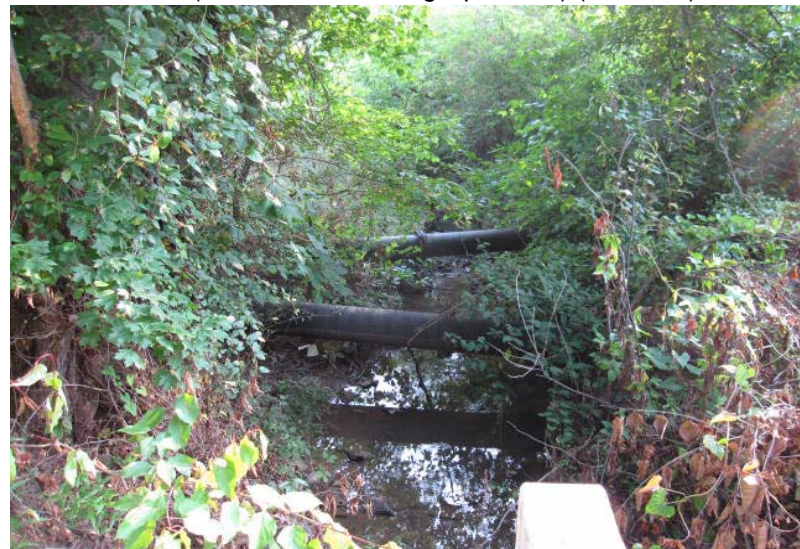
PP #6 (Sta. 6+95 – Looking Upstream) (07/17/10)
