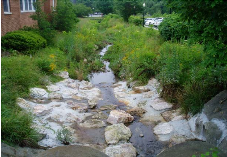
PP #1 (Sta. 0+00 – Looking Downstream) (06/14/07)
