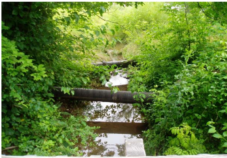
PP #6 (Sta. 6+95 – Looking Upstream) (06/14/07)
