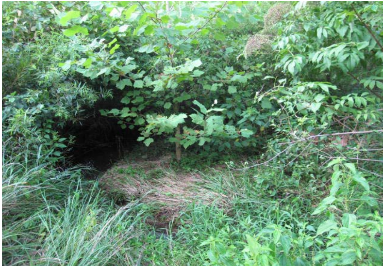
PP #4 (Sta. 4+25 – Looking Downstream) (07/17/10)
