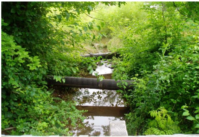
PP #6 (Sta. 6+95 – Looking Upstream) (06/14/07)
