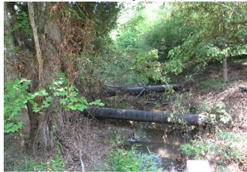
PP #6 (Sta. 6+95 – Looking Upstream) (06/10/11)
