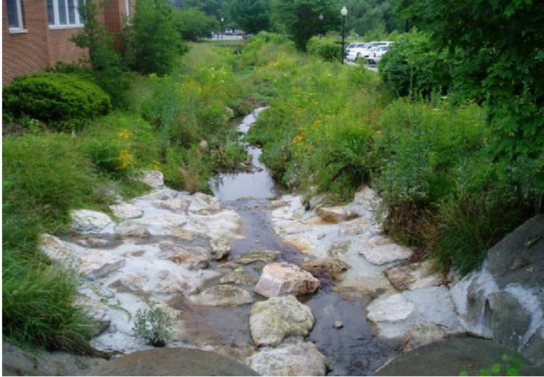
PP #1 (Sta. 0+00 – Looking Downstream) (06/14/07)
