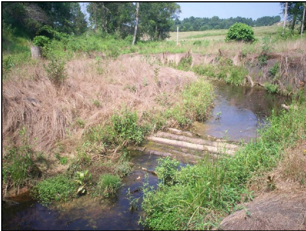
Photo 2. Log ramp structure-looking upstream.
