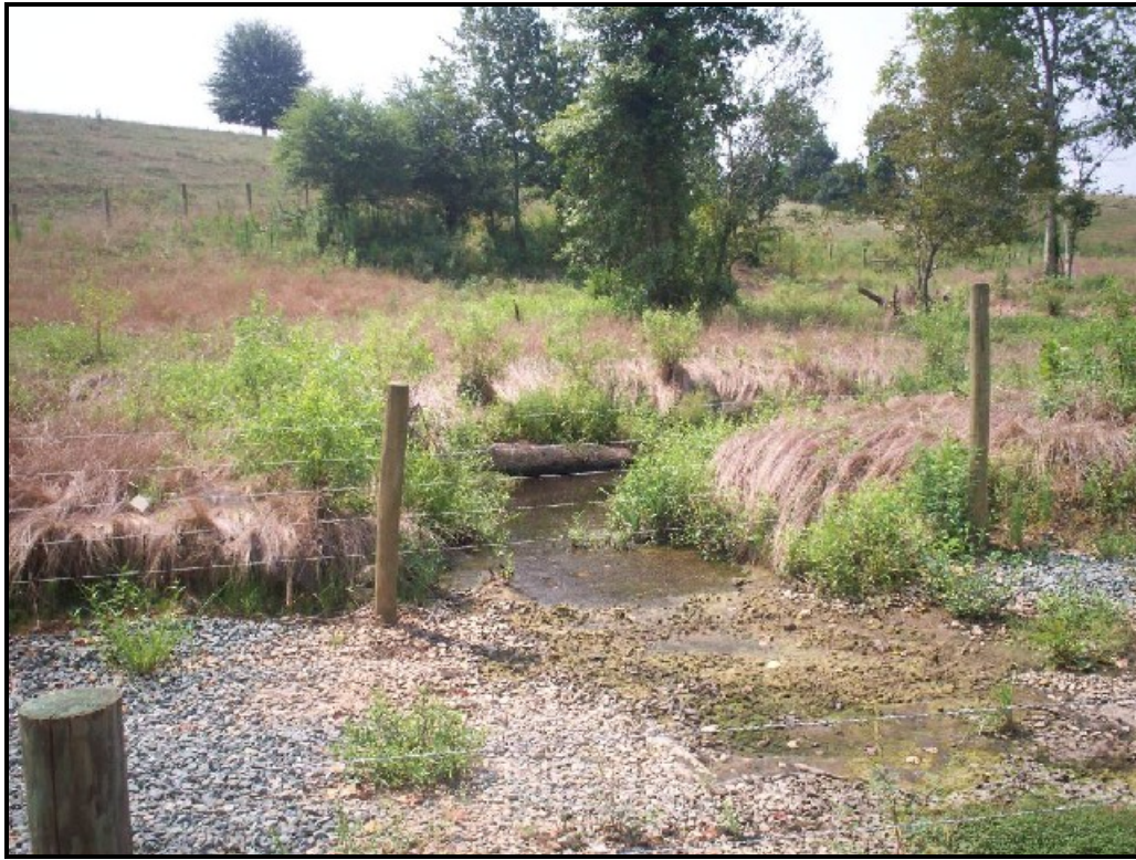
Photo 3. Ford crossing-looking downstream at log toe protection.
