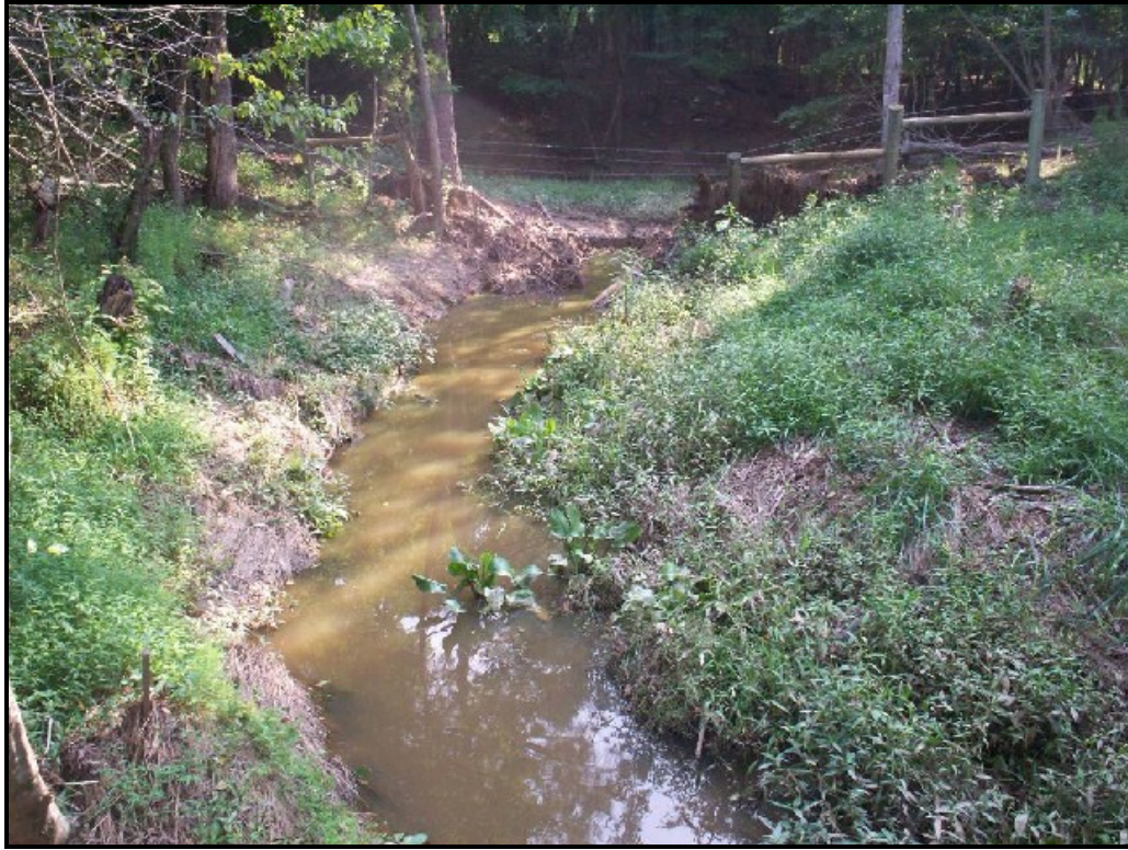
Photo 7. End of the project-looking downstream.
