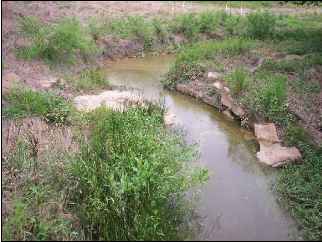
Photo 5. Stream channel; rock bank stabilization, looking upstream.
