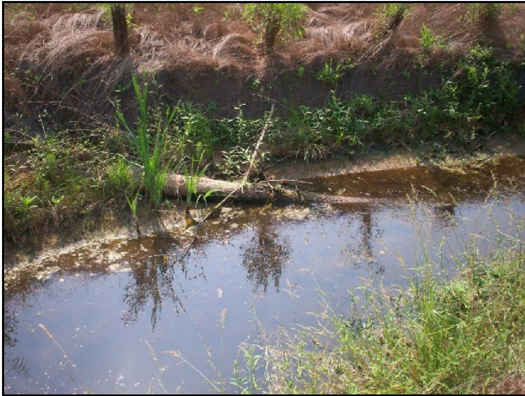
Photo 1. Log vane structure-looking downstream.
