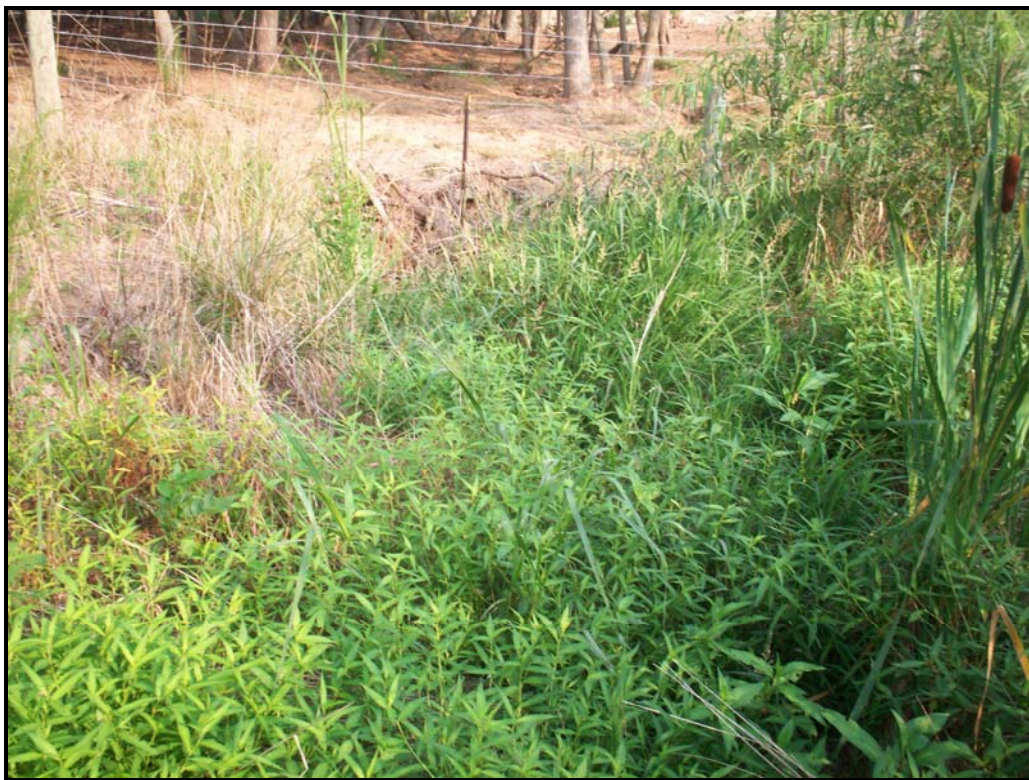
Photo 8. Upstream end of UT-2 – looking upstream; vegetation in channel.
