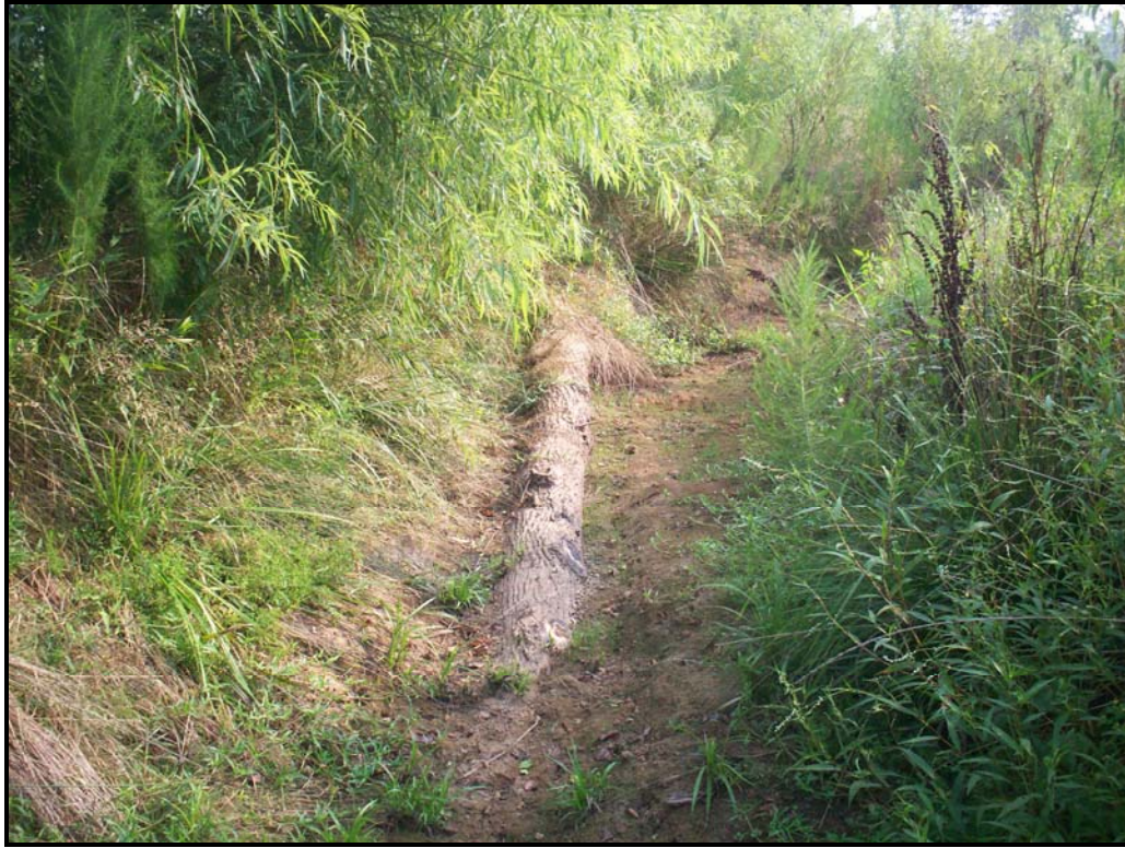
Photo 1. Log vane structure at STA 26+00 -looking downstream.
