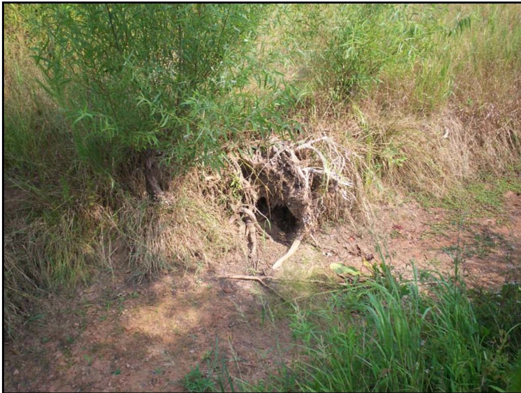
Photo 6. Rootwad on left bank at station 8+00-looking downstream.
