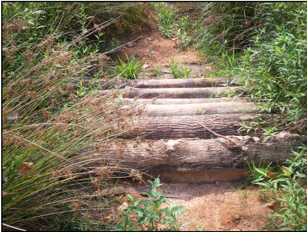
Photo 2. Log ramp structure at station 10+90 - looking downstream.
