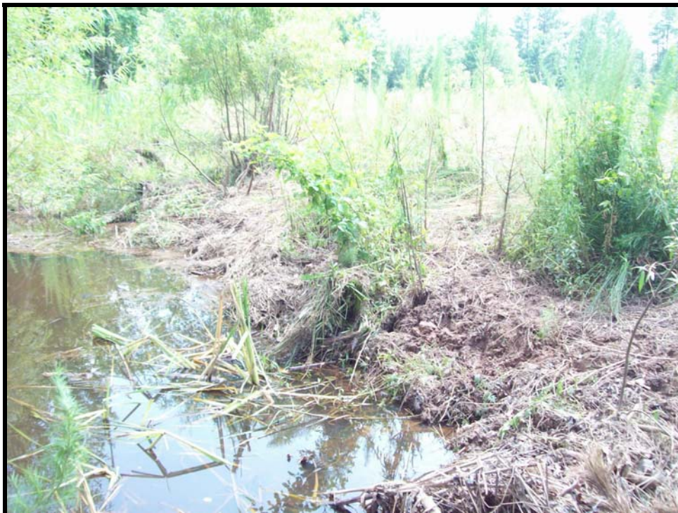
SPA 11. Erosion on left bank due to cattle at Station 49+50.
