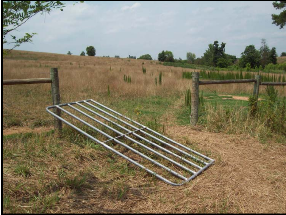
SPA 10. Cattle gate off hinges at Station 49+00.
