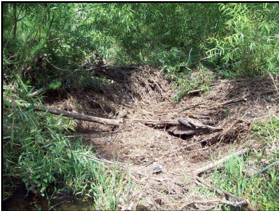
SPA 4. Debris jam caused by fallen tree blocking water flow at Station 46+50.
