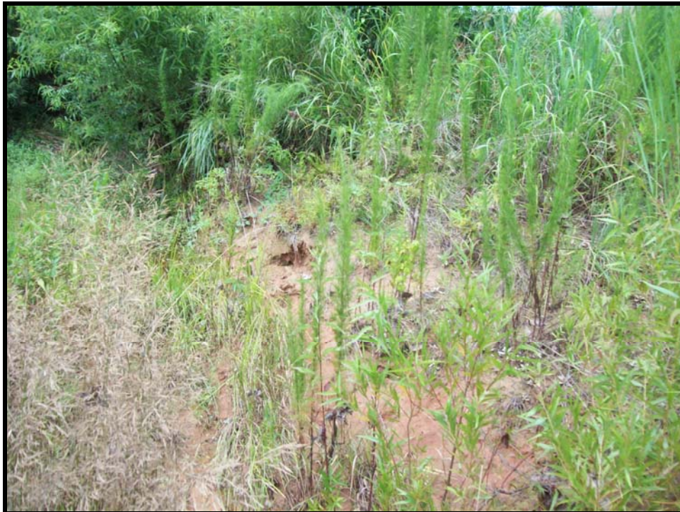
SPA 2. Minor erosion on left bank at Station 34+00.
