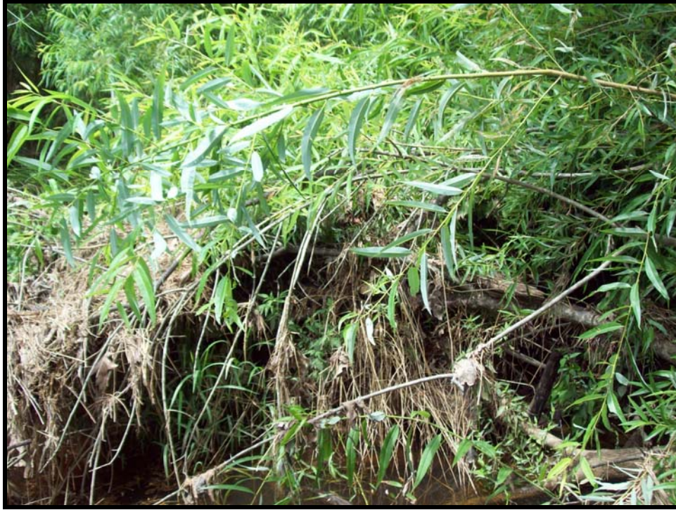
SPA 1. Debris jam at Station 32+50.
