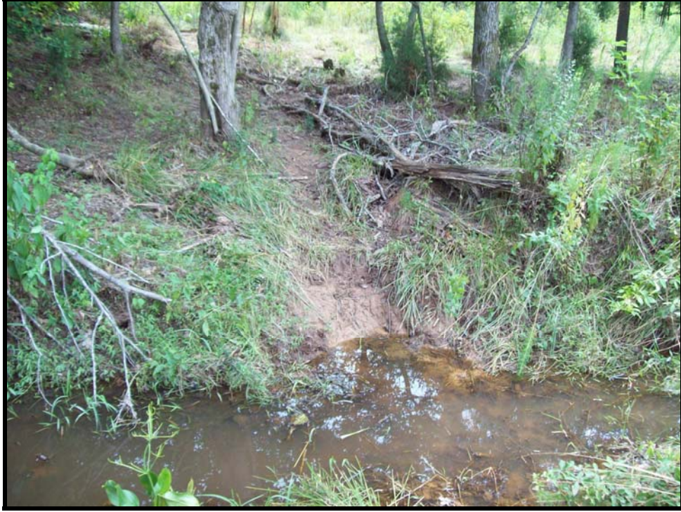
SPA 12. Erosion on right bank due to cattle hoof shear at Station 53+00.
