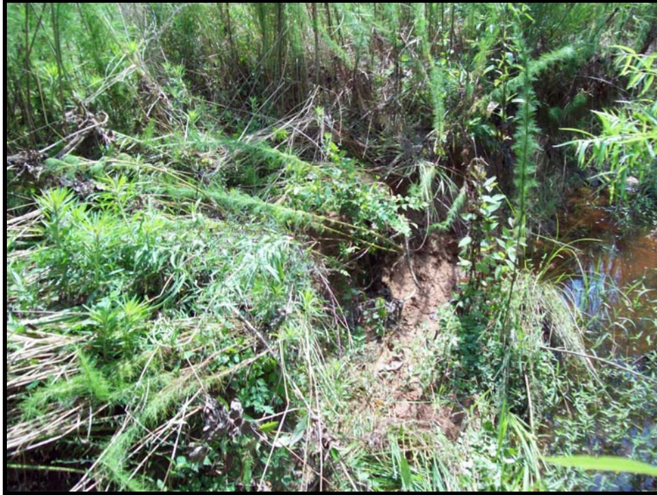
SPA 3. Minor erosion on right bank at Station 40+25.
