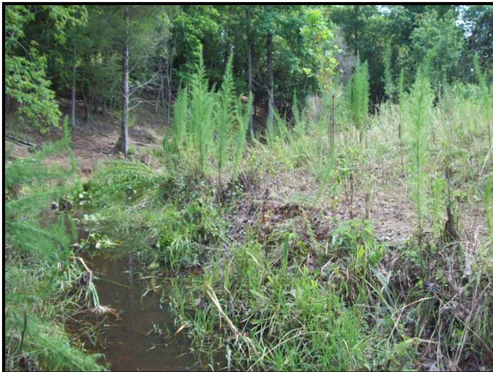
SPA 8. Severe damage to vegetation and bank erosion caused by cattle within easement from Station 48+50 to 56+75.
