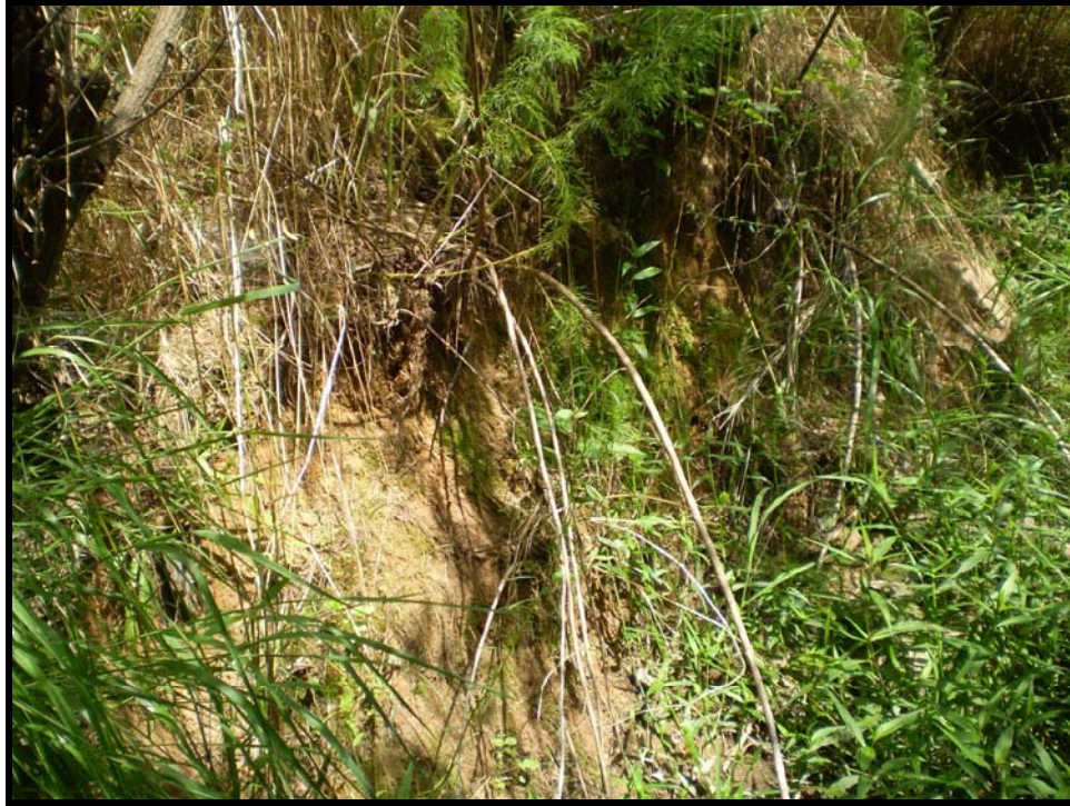
SPA 5 – Minor right bank erosion, UT1 Sta. 40+10 to 40+50.
