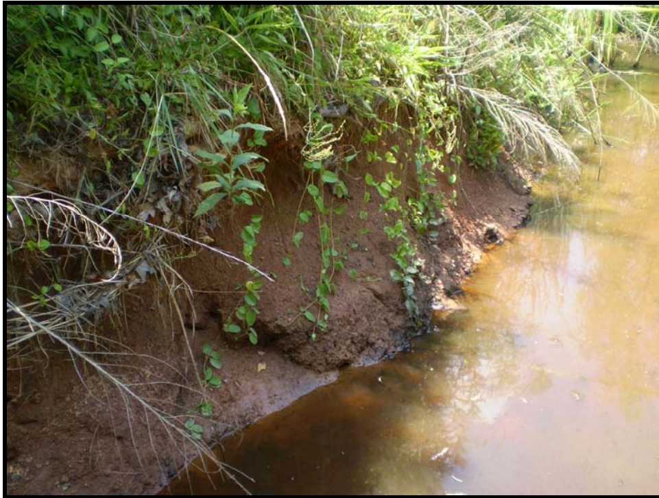
SPA 4 – Minor left bank erosion, UT1 Sta. 44+60 to 45+10.
