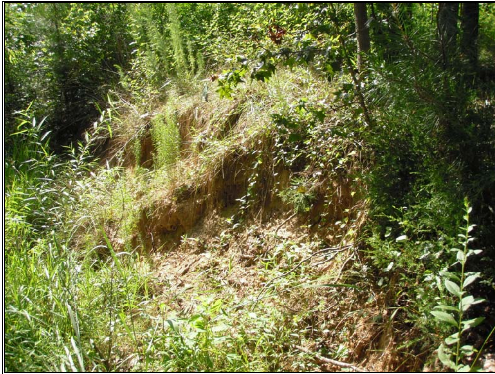
SOA 2 – Minor right bank erosion, UT1 Sta. 47+50 to 47+80.
