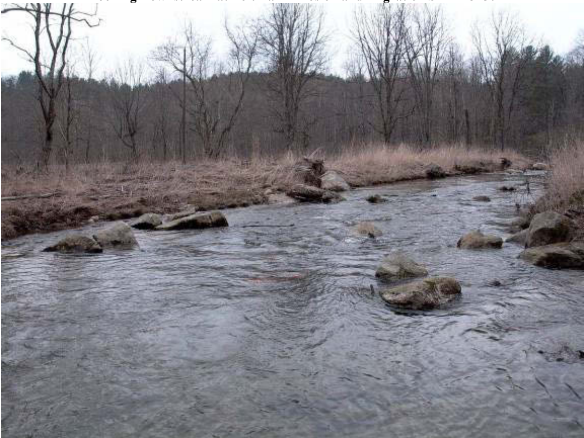
Looking Downstream at Boulder Clusters STA ~ 11+50
