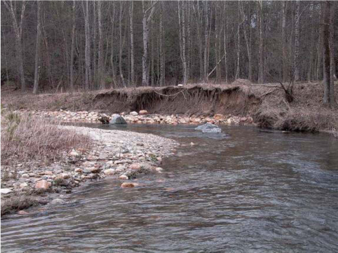
Looking Downstream at Right Bank Erosion and Migration STA ~ 32+50
