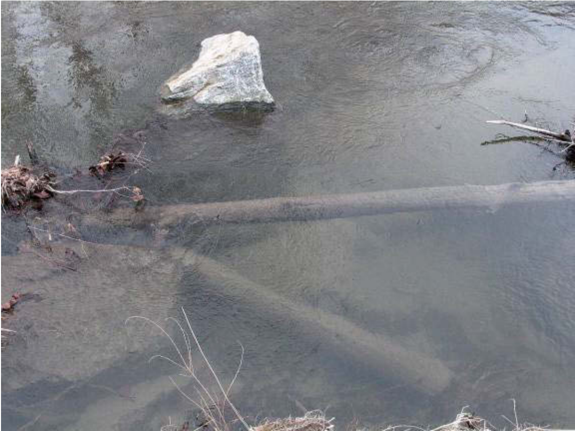
Exposed Root Wads and Boulder Toe Right Bank STA ~6+00
