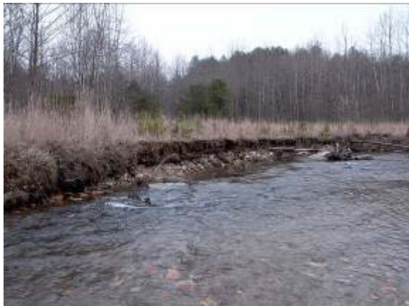
Issue Photo 1. Bank Erosion STA ~28+75 Reach 2
