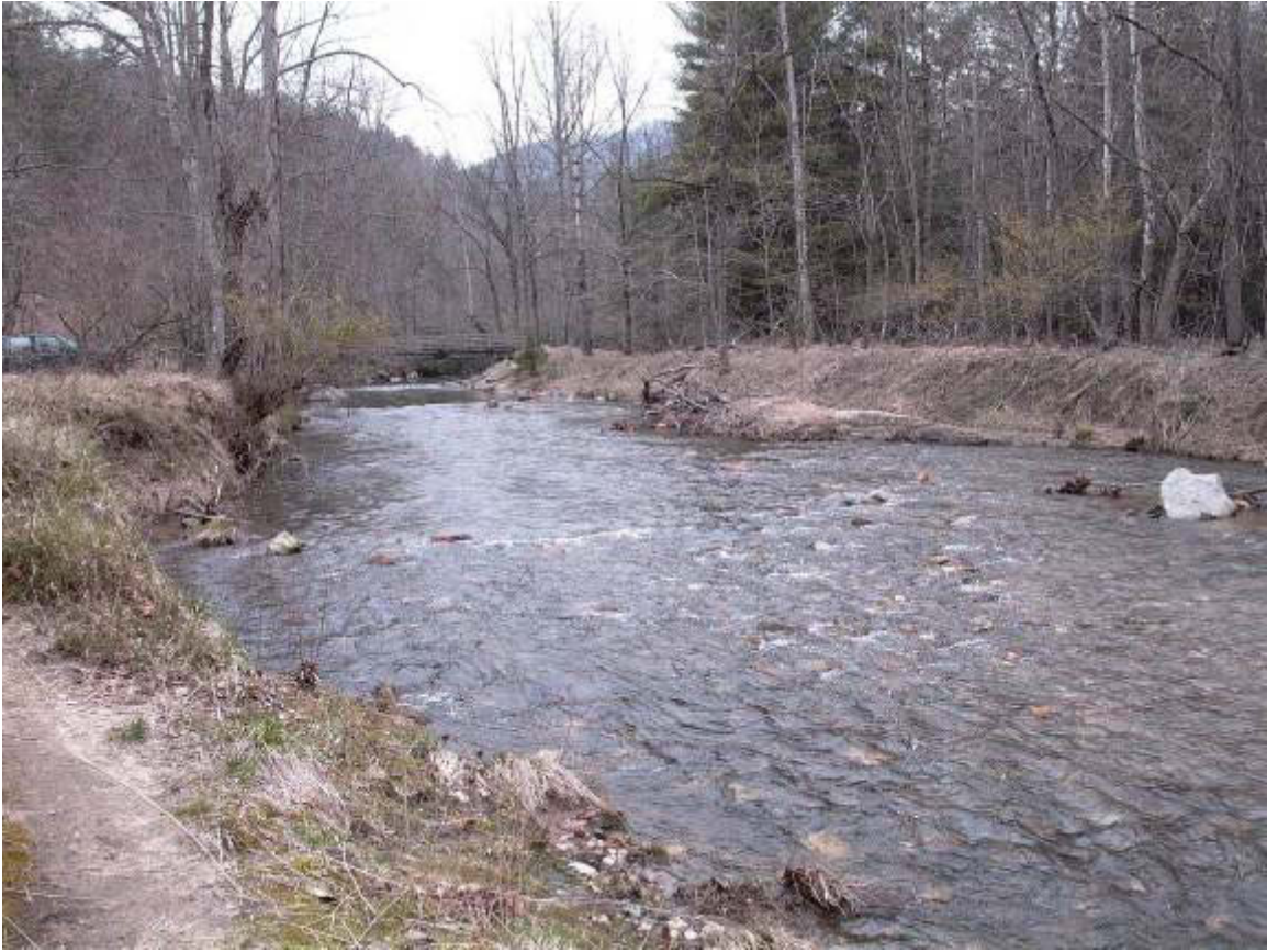
Looking Upstream STA~ 2+50
