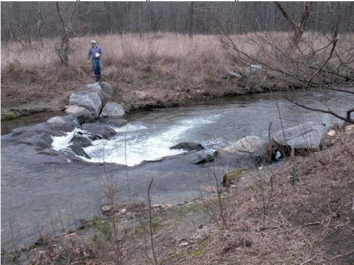
Looking Downstream at Rock Cross Vane STA~ 11+00
