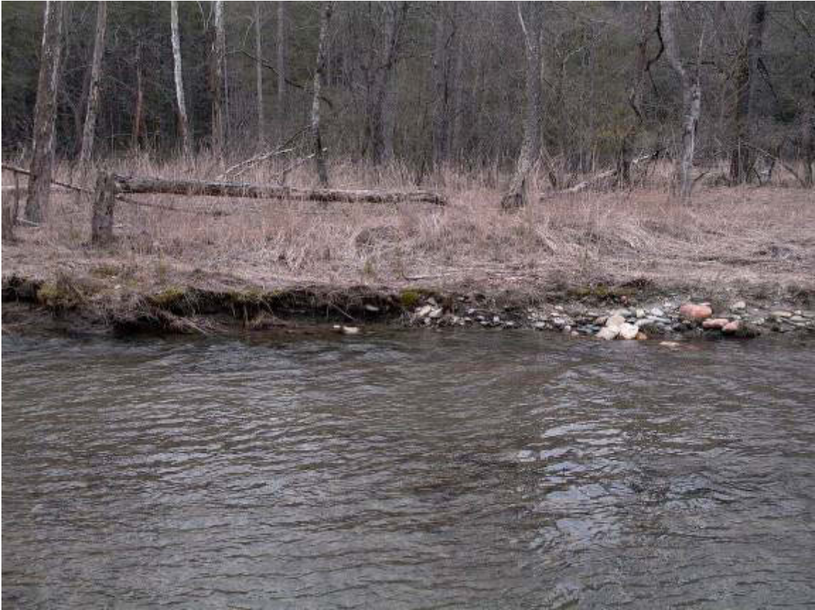
Looking Downstream at Left Bank Erosion STA ~ 5+00
