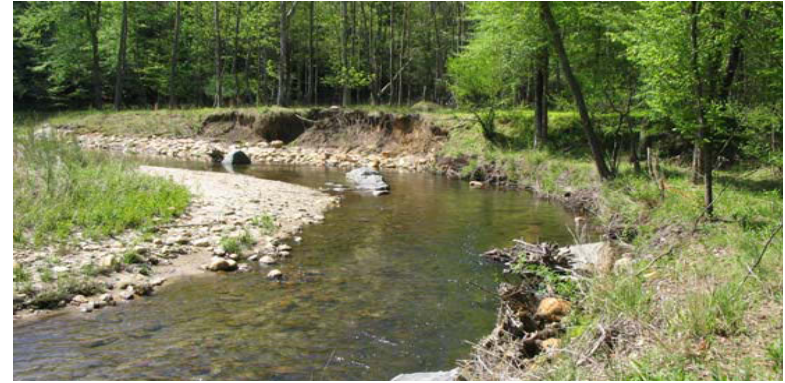
Photo of Cross-Section 7 - Reach 4 - Looking Downstream @ STA 32+70
