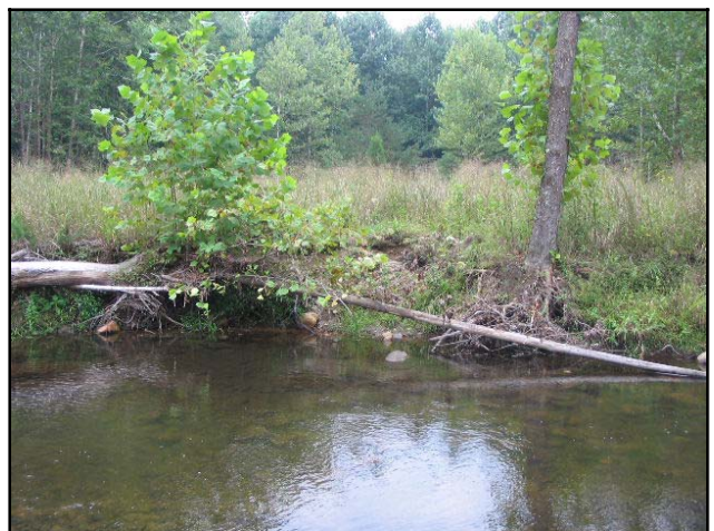
PA 31 Failed Log J-Hook Left Bank Erosion and Migration STA 29+50
