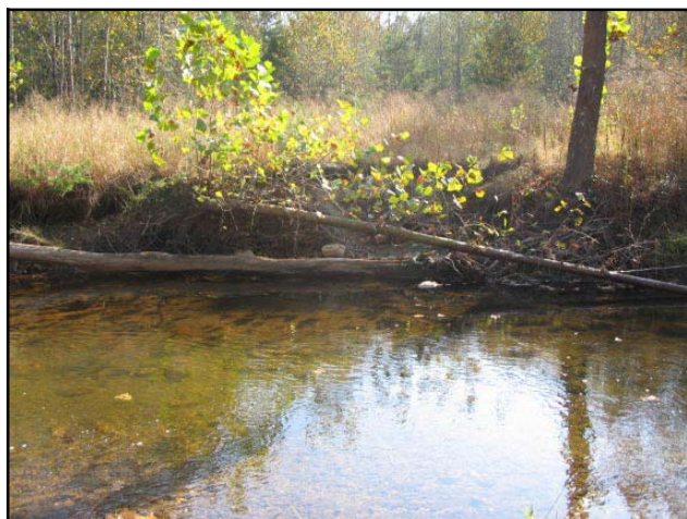
PA 32 Left Bank Erosion and Migration STA 29+75
