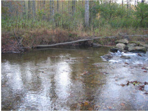
PA10 Left Bank STA 11+25 Erosion Behind Vane
