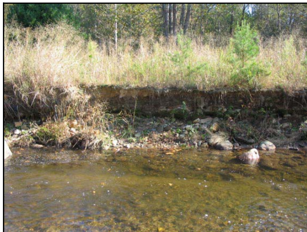
PA 31 Failed Log J-Hook Left Bank Erosion and Migration STA 29+50
