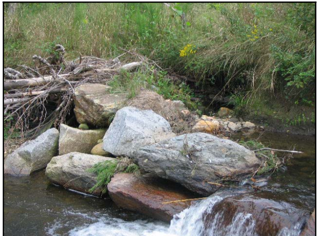
PA 28 Failed Rock Cross Vane Piping Behind Right Vane Arm STA 25+00
