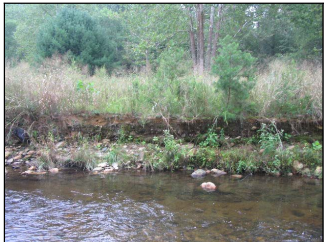
PA 31 Failed Log J-Hook Left Bank Erosion and Migration STA 29+50
