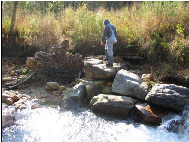
PA 28 Failed Rock Cross Vane Piping Behind Right Vane Arm STA 25+00
