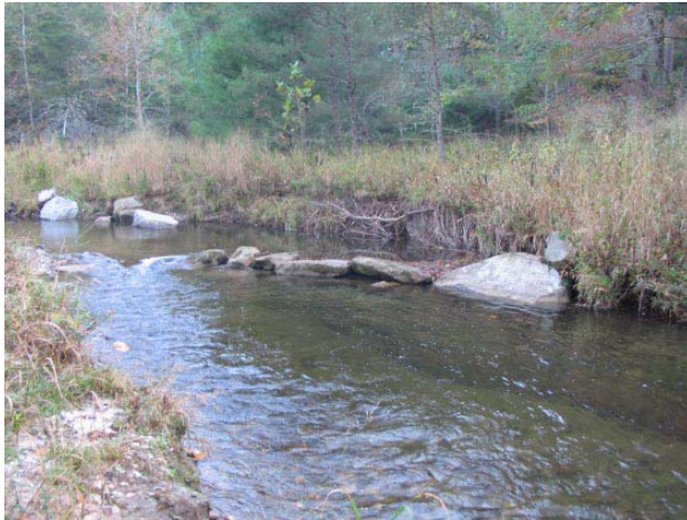
PA7 Looking Upstream STA 10+75 at J-hook and Left Bank Erosion
