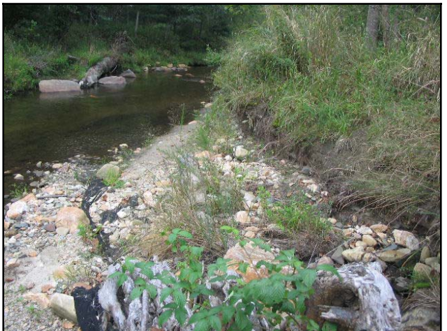
PA 28 Failed Rock Cross Vane Piping Behind Right Vane Arm STA 25+00
