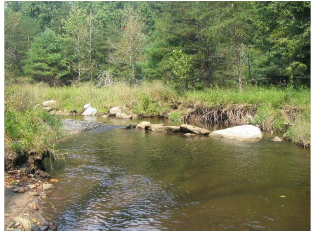
PA7 Looking Upstream STA 10+75 at J-hook and Left Bank Erosion
