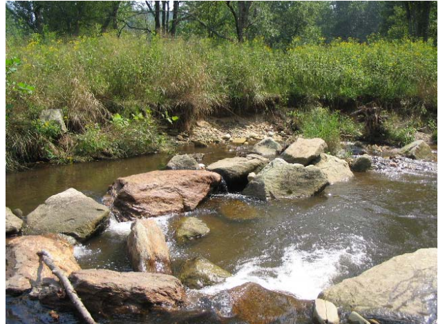
PA 13 Looking Downstream STA 13+00 Bank Erosion and Piping around Structure Arm
