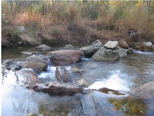
PA 13 Looking Downstream STA 13+00 Bank Erosion and Piping around Structure Arm
