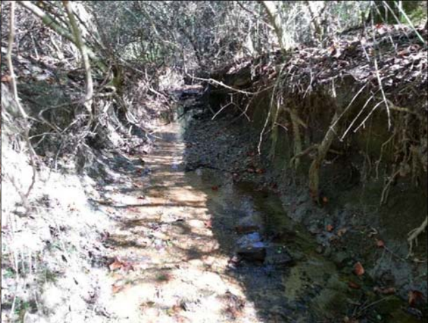
Photo 8: View of accelerated erosion and undercut banks on Stony Fork.
