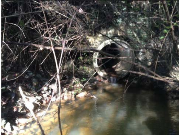
Photo 1: Head of project at exit from culvert at Federal Rd.
