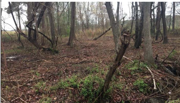
Photo 5: Near top of T2 showing mechanical removal of privet that occurred in December 2017.
