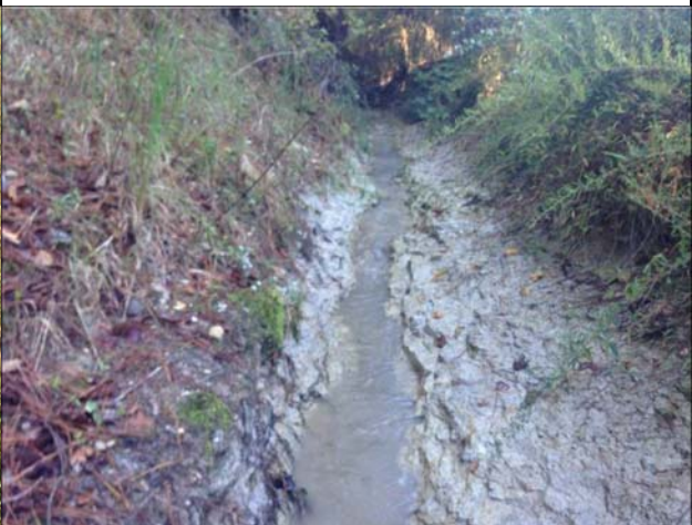
Photo 6: View of clay channel bottom on Stony Fork along channelized stream.
