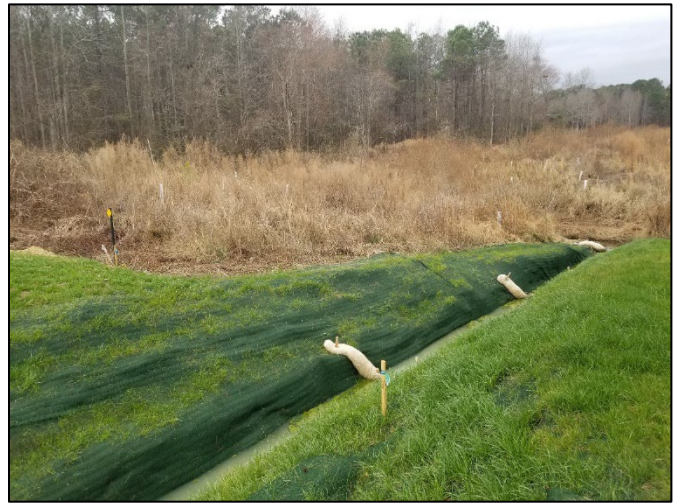
Easement Encroachment Area – 2/24/22
