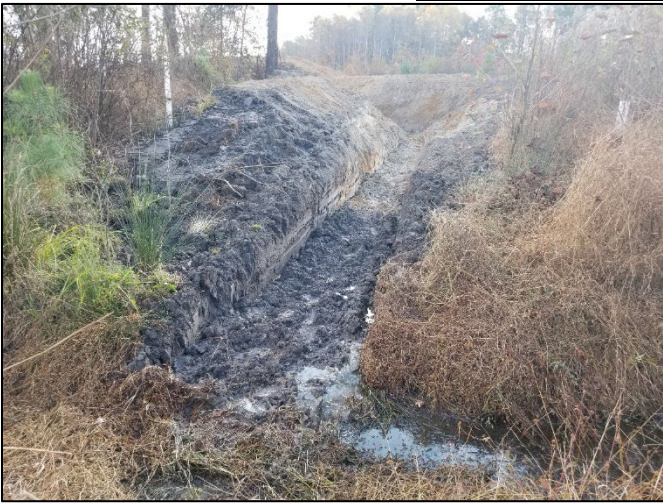
Easement Encroachment Area – 11/19/21
