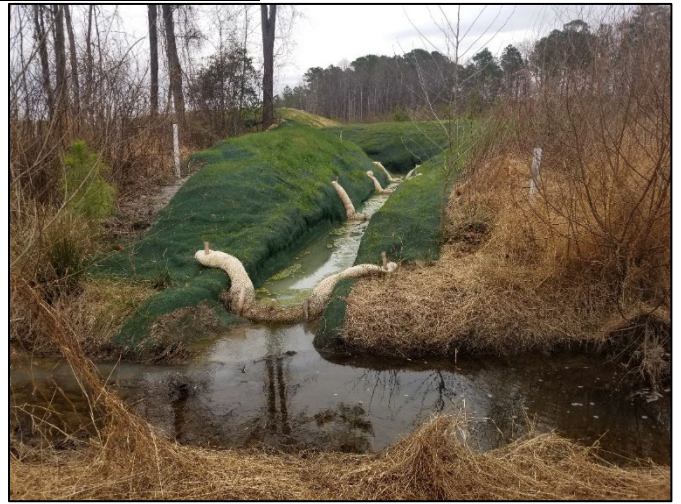
Easement Encroachment Area – 2/24/22
