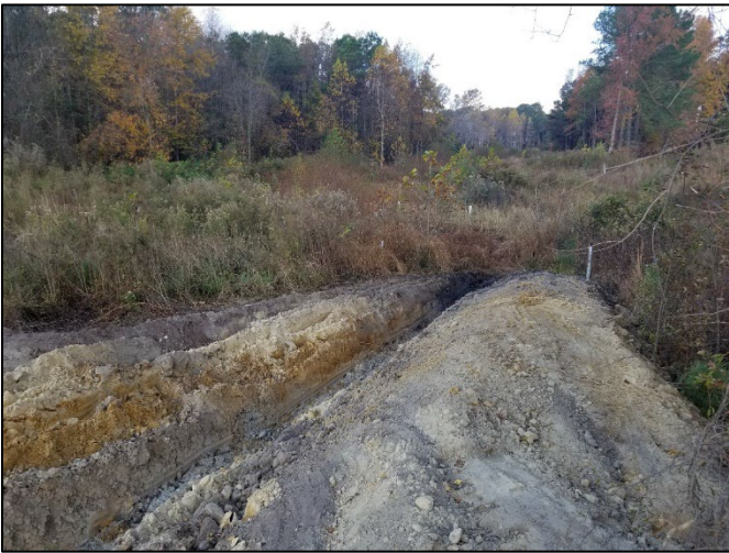
Easement Encroachment Area – 11/19/21
