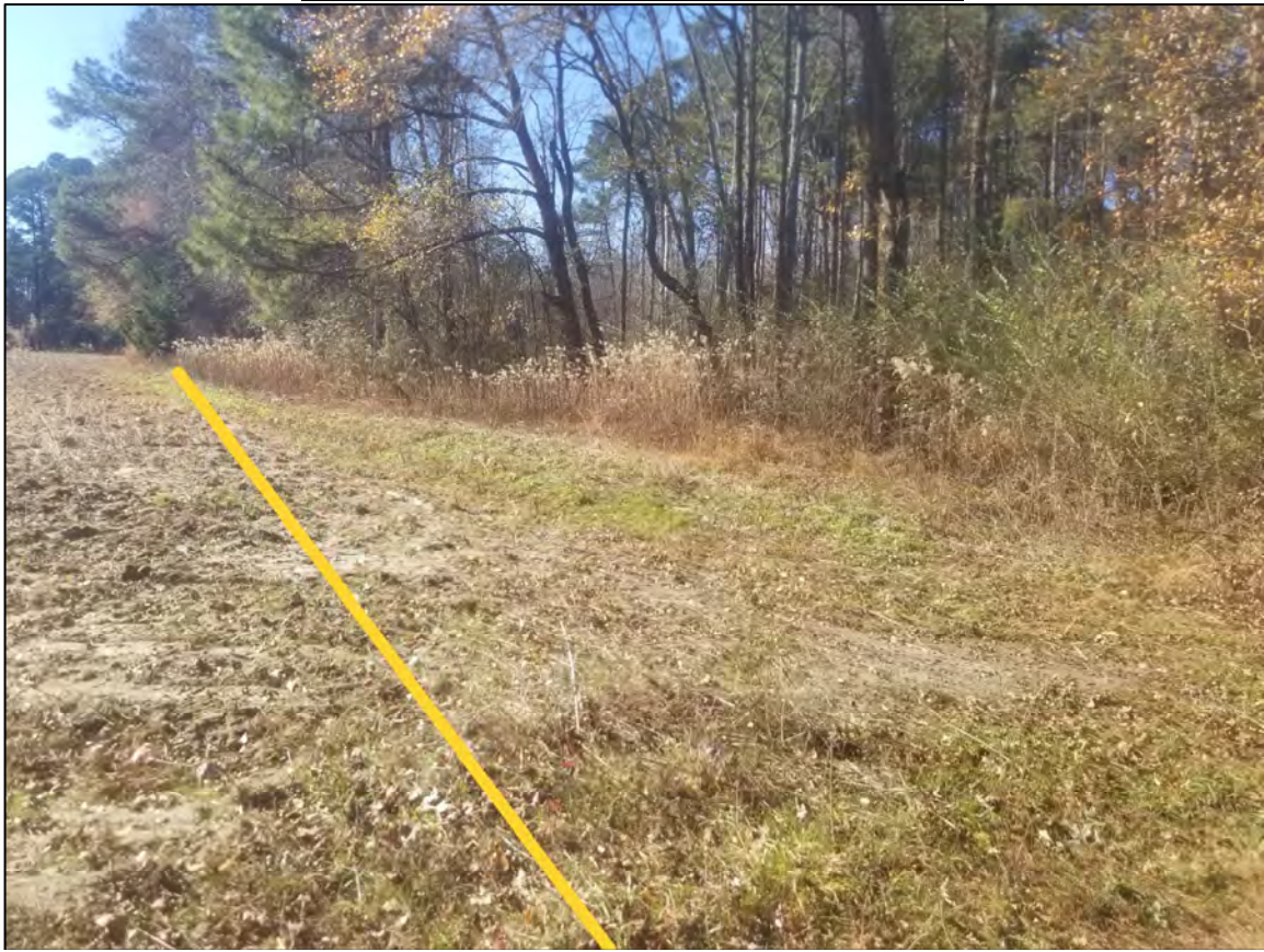
Scalping near the bottom of the site, with approximate easement line – 12/7/23
