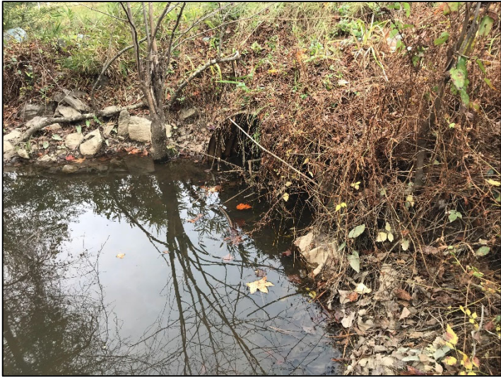
DOT Culvert at Brogden Rd. (Entrance) (11/16/2022)
