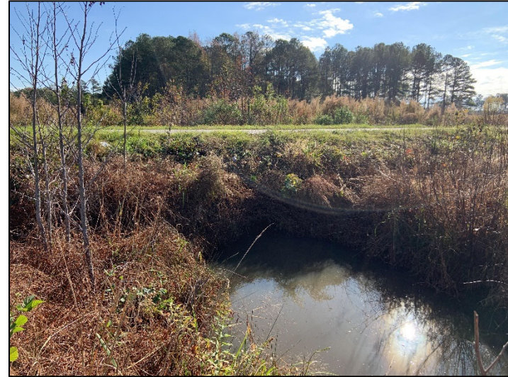
DOT Culvert at Yelverton Grove Rd. (Exit) (11/16/2022)
