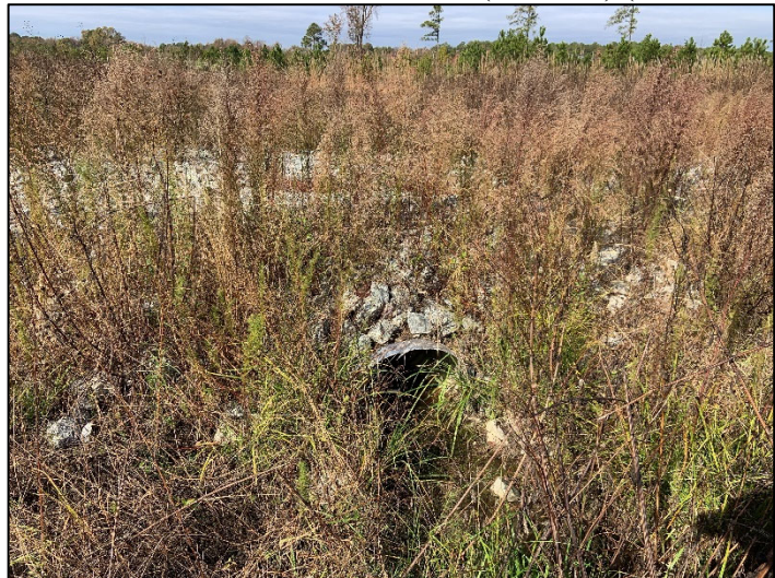
Culvert at JH1-B Crossing (Entrance) (11/16/2022)
