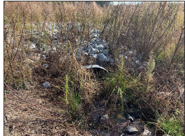
Culvert at JH1-B Crossing (Exit) (11/16/2022)
