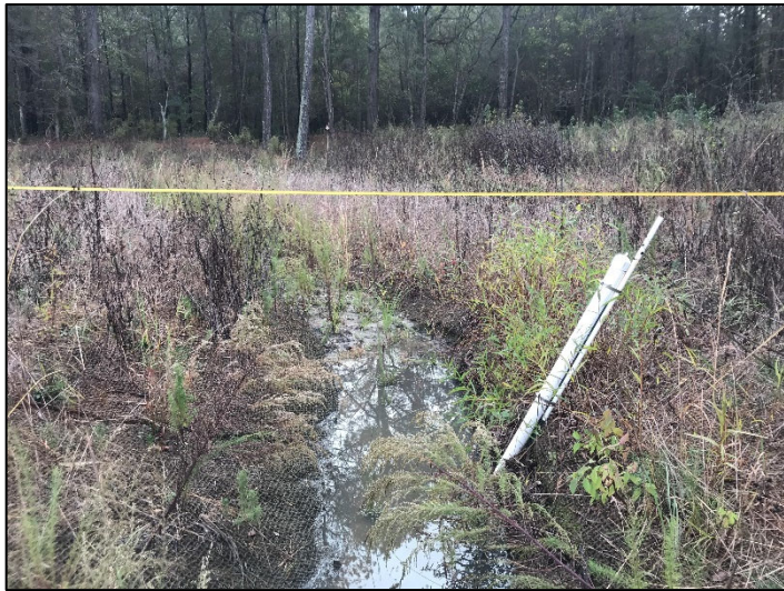
Hay bale toe with live stakes at JH1-A flow gauge (11/16/2022)
