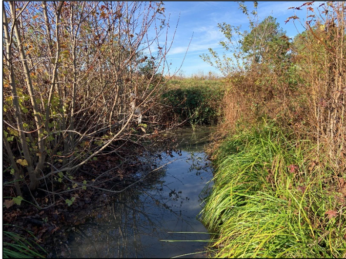
DOT Culvert at Yelverton Grove Rd. (Entrance) (11/16/2022)
