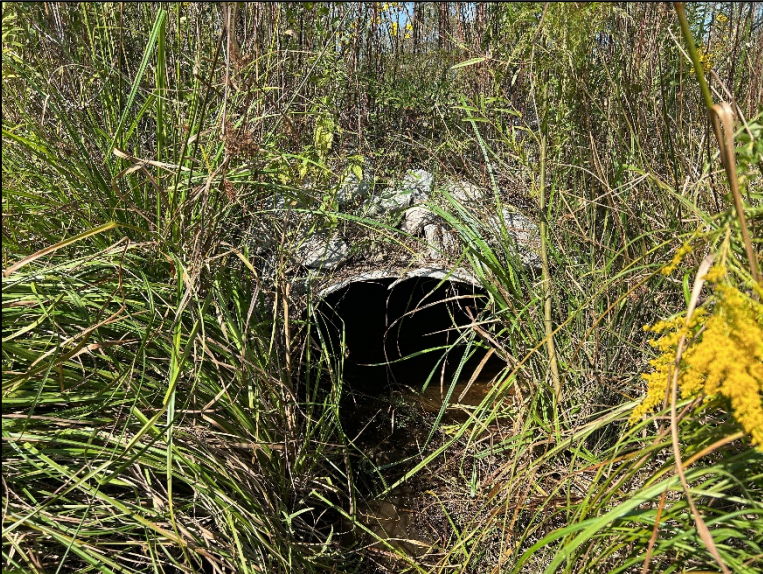
PP-8 Culvert at JH1-B Crossing (Entrance) (10/3/2023)
