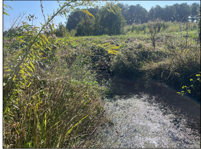
PP-7 DOT Culvert at Yelverton Grove Rd. (Exit) (10/3/2023)
