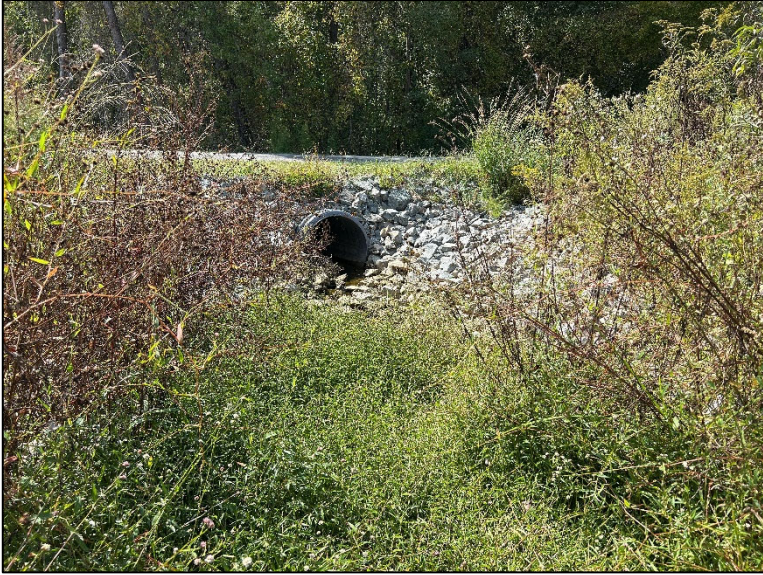
PP-10 New DOT Culvert at Brogden Rd. (Entrance) (10/3/2023)
