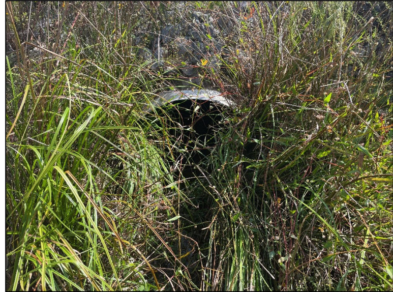
PP-9 Culvert at JH1-B Crossing (Exit) (10/3/2023)
