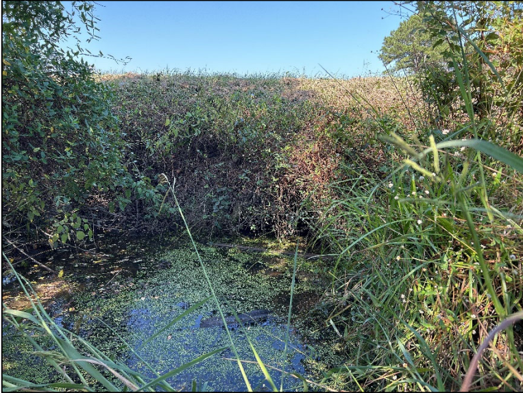
PP-6 DOT Culvert at Yelverton Grove Rd. (Entrance) (10/3/2023)
