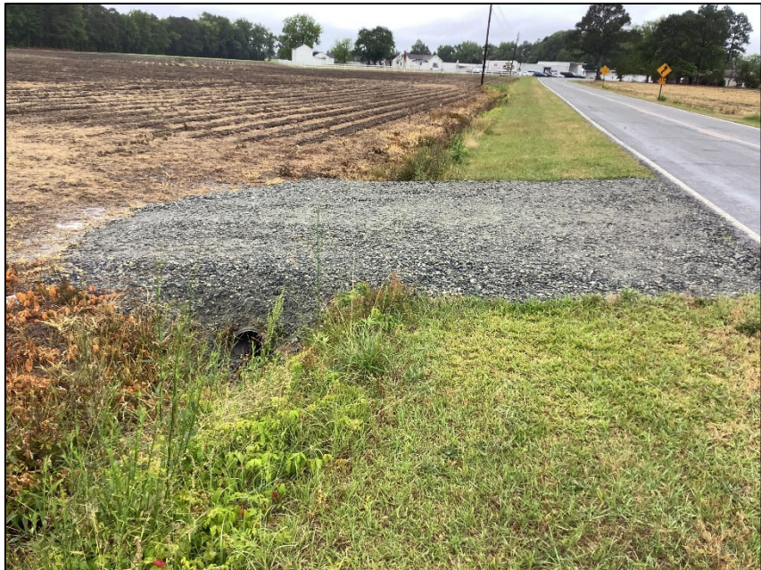
Newly installed agricultural driveway near JH2 (5/19/2023)
